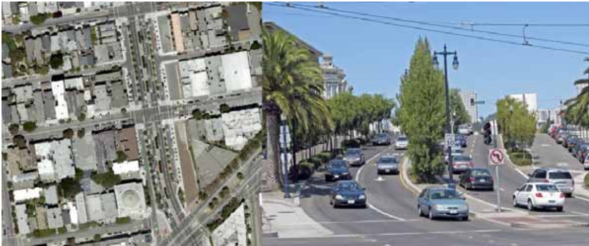
The boulevard replacing San Francisco’s Central Freeway is approx. 125’ wide.
