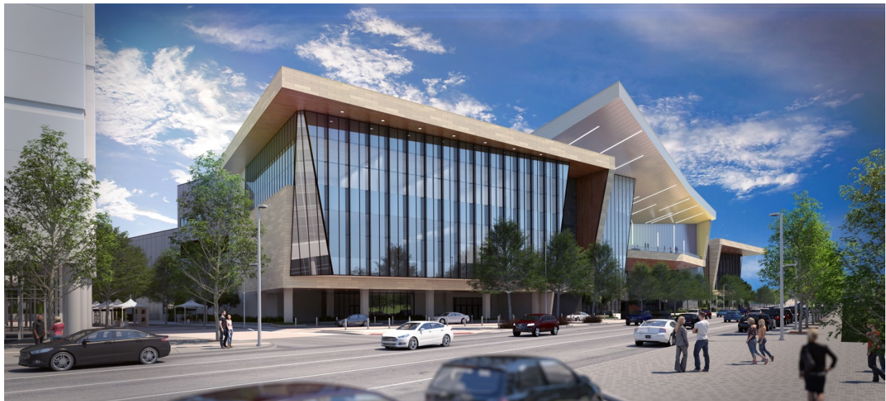
Figure 1: West façade of the Downtown Convention Center facing Robinson Avenue
