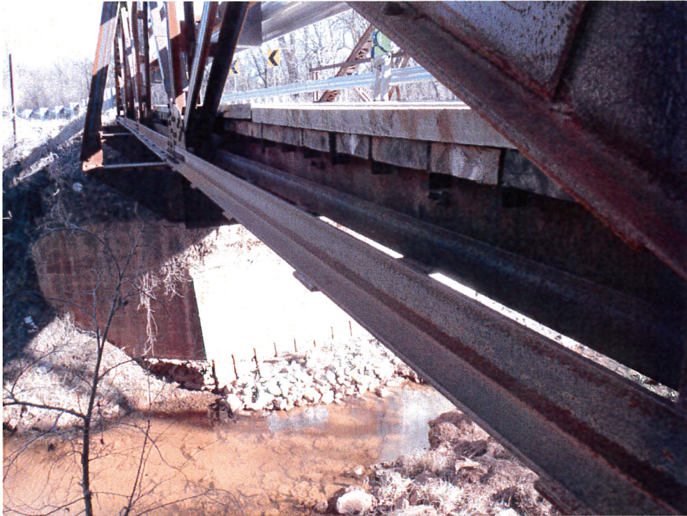
Figure 9: New Members of LC West Truss
