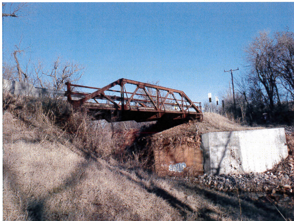
Figure 16: Old North Abutment and New Retaining Wall
