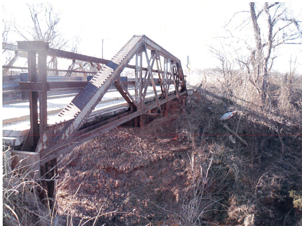
Figure 8: Typical Condition of Truss
