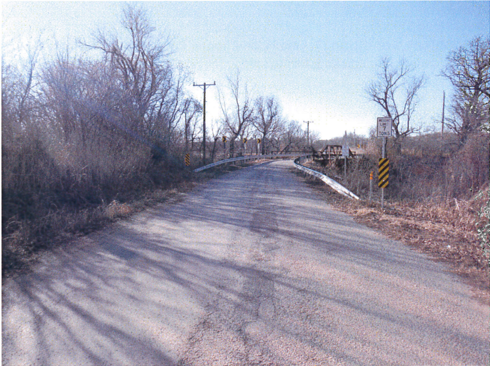
Figure 1: Bridge from North Approach
