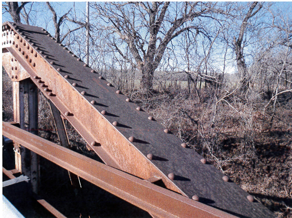
Figure 12: Bridge Rail welded to Truss Members
