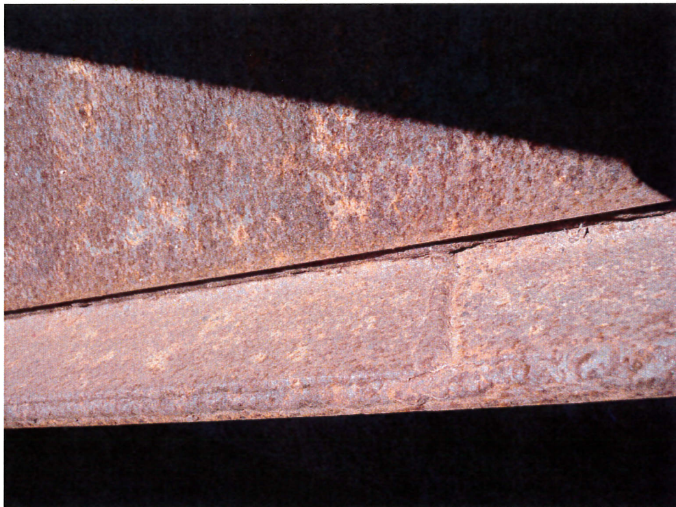
Figure 10: Repair of West Truss End Post at South Abutment
