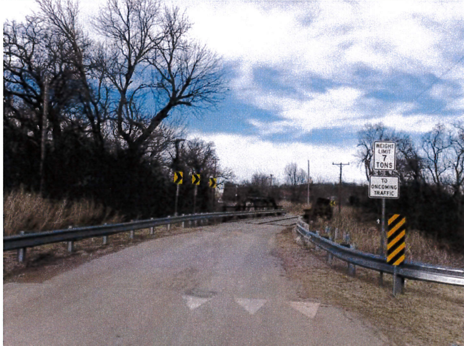
Photograph 3 - Looking north at 7-ton load posting sign at south approach.
