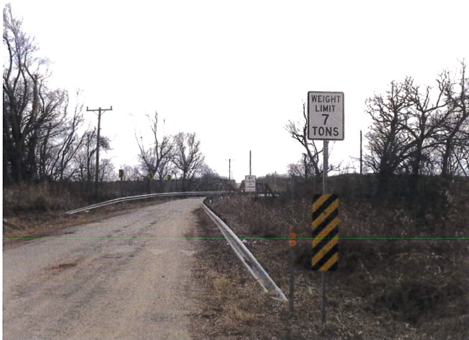
Photograph 4 - Looking south at 7-ton load posting sign at north approach. Note: The northeast bridge marker is laying on the ground.
