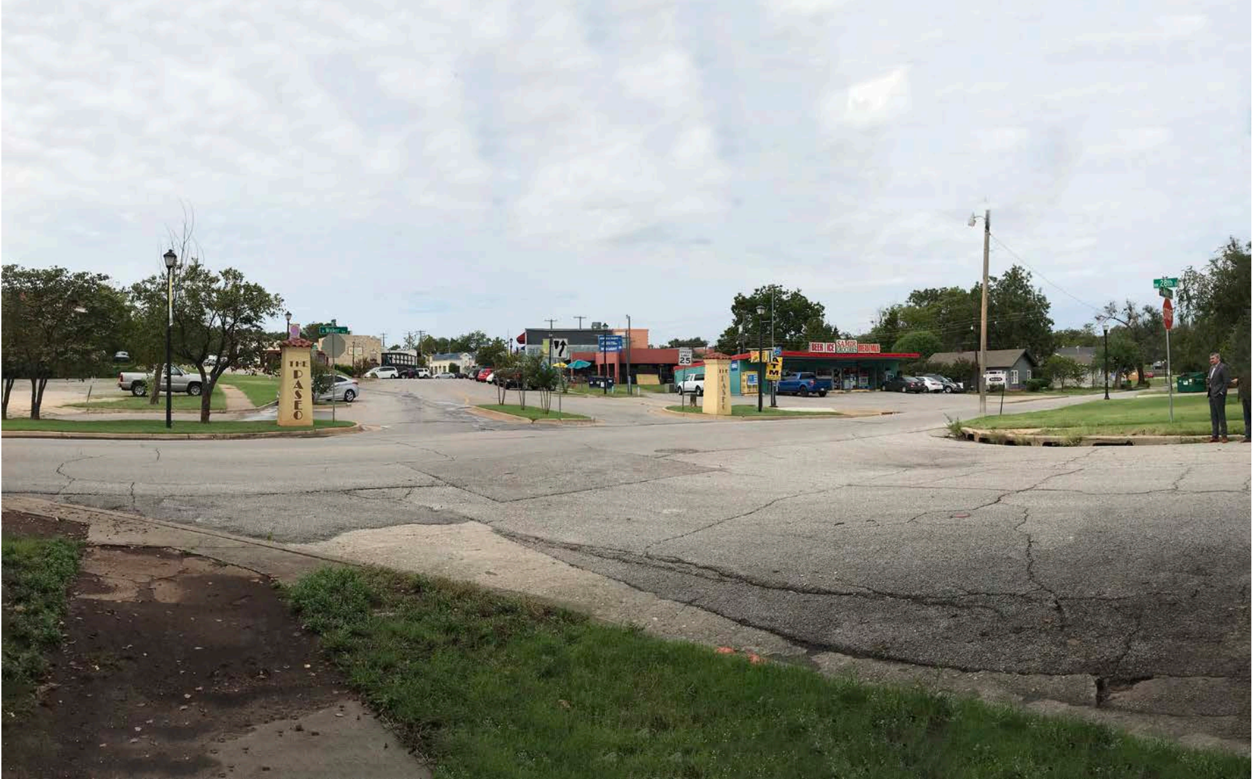
Figure 24. Intersection of Paseo, Walker Avenue and NW 28th Street. This wide intersection, an important entry into the Paseo District, frequently floods, and facilitates speeding north-south on Walker Avenue. The intersection lacks pedestrian crossings, and the sidewalks are in disrepair.
