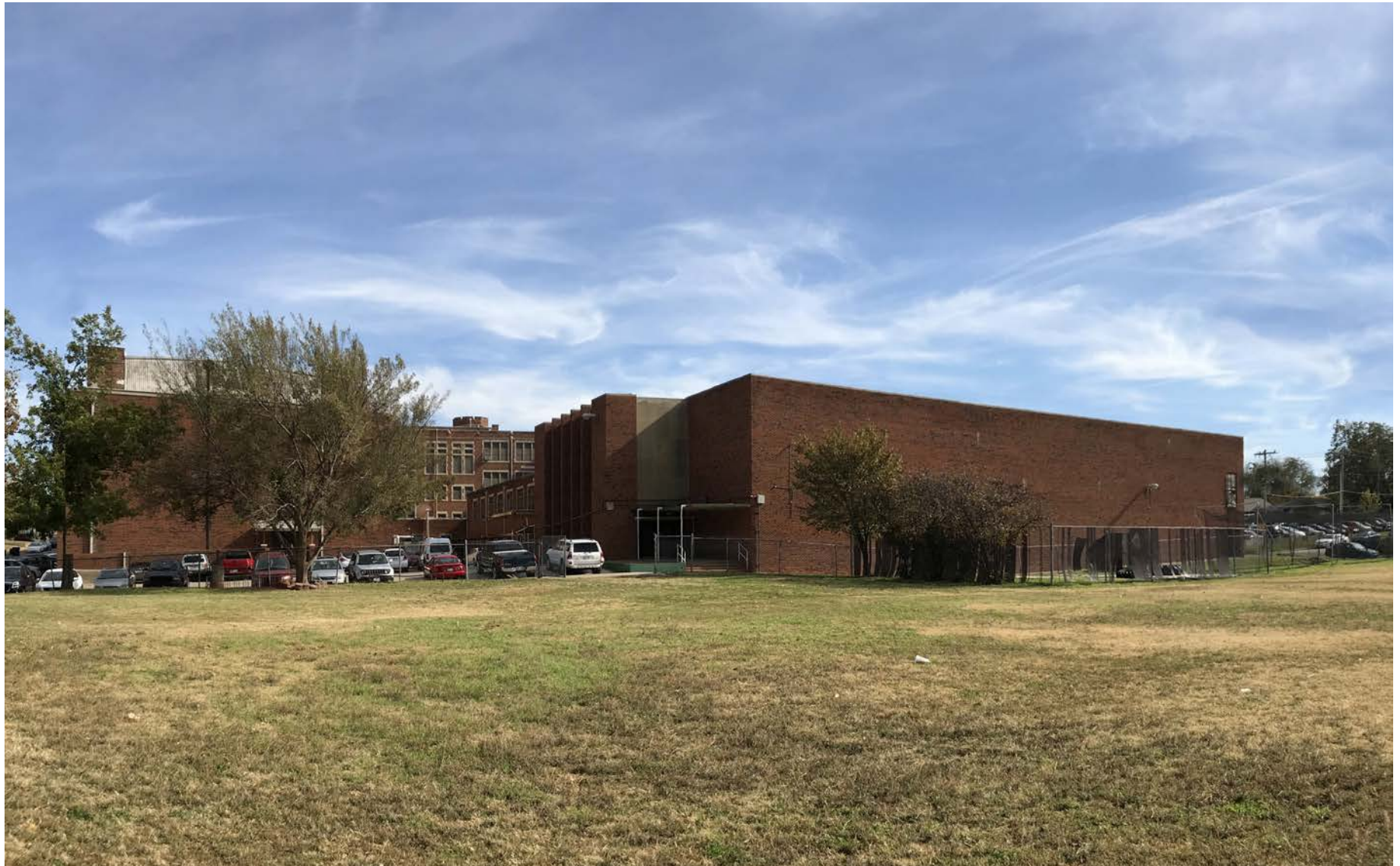
Figure 29. A view of Harding from the athletic field. The large impervious footprint of the school and adjacent parking structures, as well as the steep grade changes of surrounding blocks, creates more stormwater runoff than the current drainage infrastructure can handle. The volume causes flooding inside the school and on surrounding streets.
