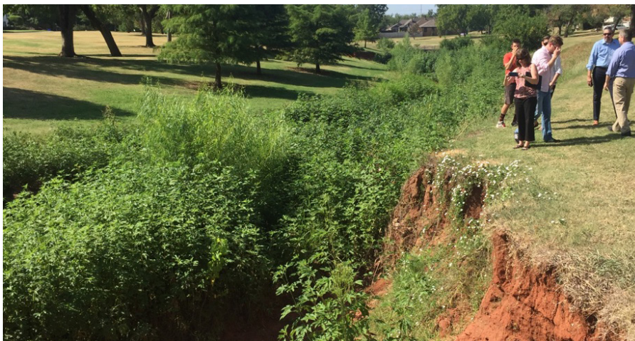
Figure 15. The sides of Guy James Creek have eroded, forming steep banks.
