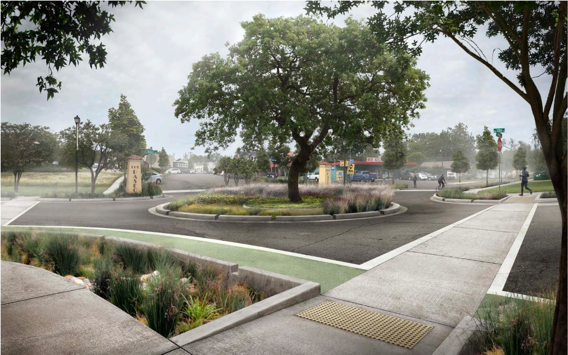
Figure 25. A recessed roundabout slows vehicles moving through the intersection and captures stormwater during rain events. New sidewalks and street markings improve pedestrian safety, dedicated bike lane address cyclist safety, and planted bump-outs collect and infiltrate additional street runoff.
