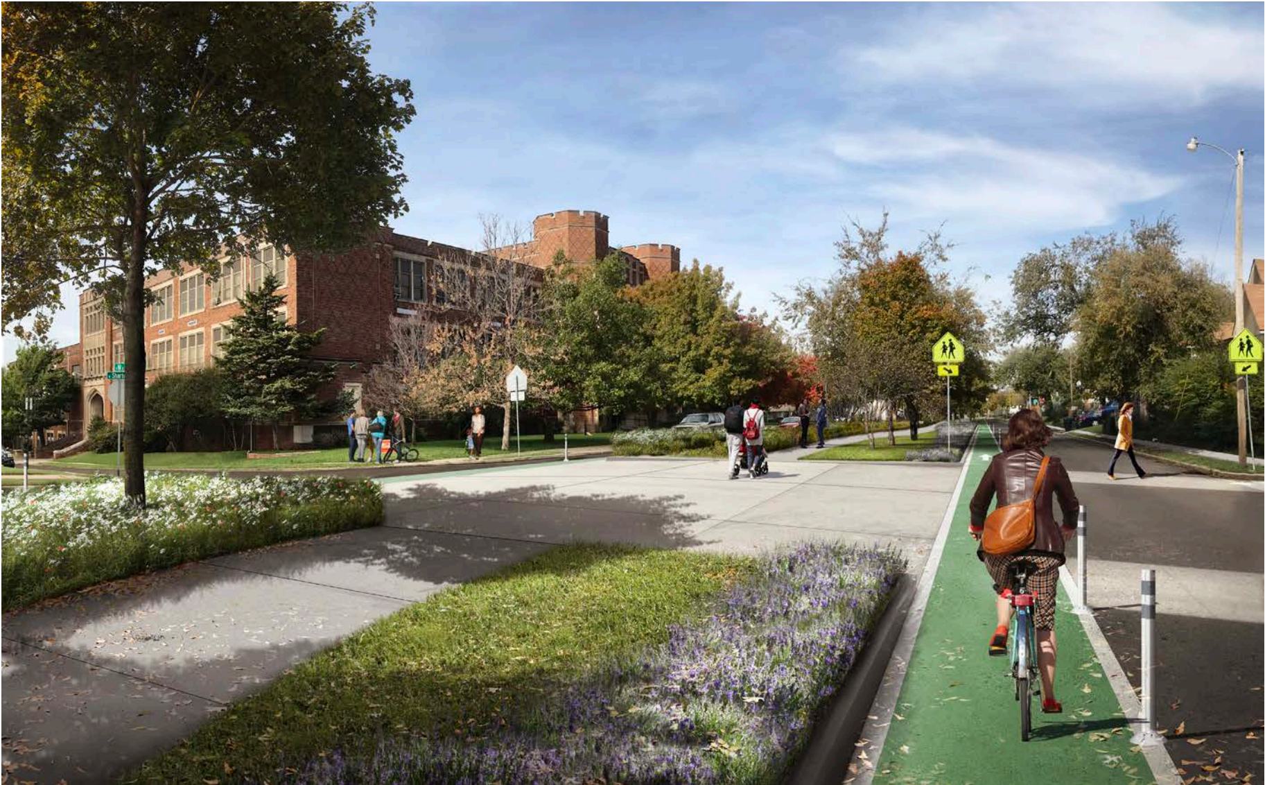
Figure 40. A speed table and well-marked crosswalks slow traffic at the intersection of Hill and Shartel Avenue. A path through the medians provides a continuous route for pedestrians, and separated bike lanes improve safety for bicyclists.
