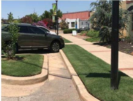
Figure 9. Large drainage channels increase the speed of water along Paseo and create trip hazards for pedestrians.
