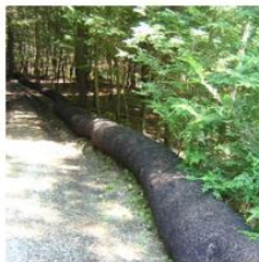
RUNOFF DIVERSION View »
