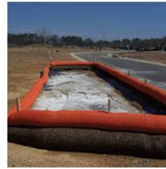
CONCRETE WASHOUT View »
