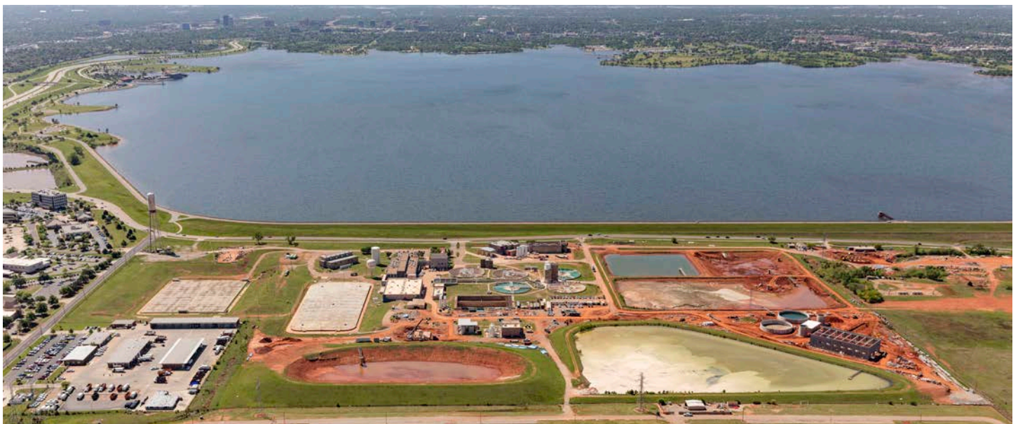
Figure 12: Hefner water treatment plant
