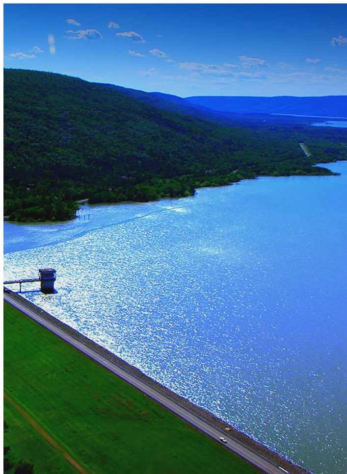
Figure 11: Sardis Reservoir, Photo courtesy Water Unity Oklahoma
