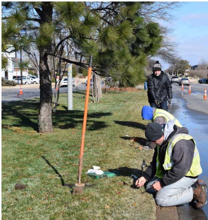
Figure 29: Median retrofit project on Classen Boulevard
