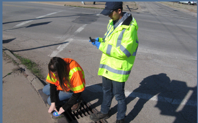
Storm drain marker installation
