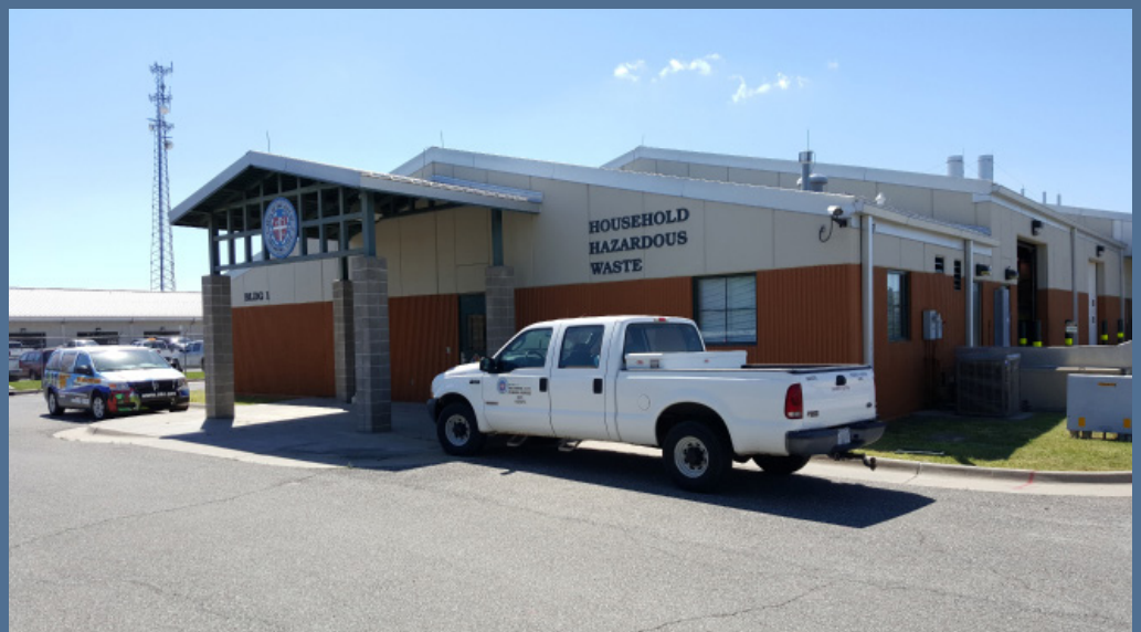
Household Hazardous Waste Facility
