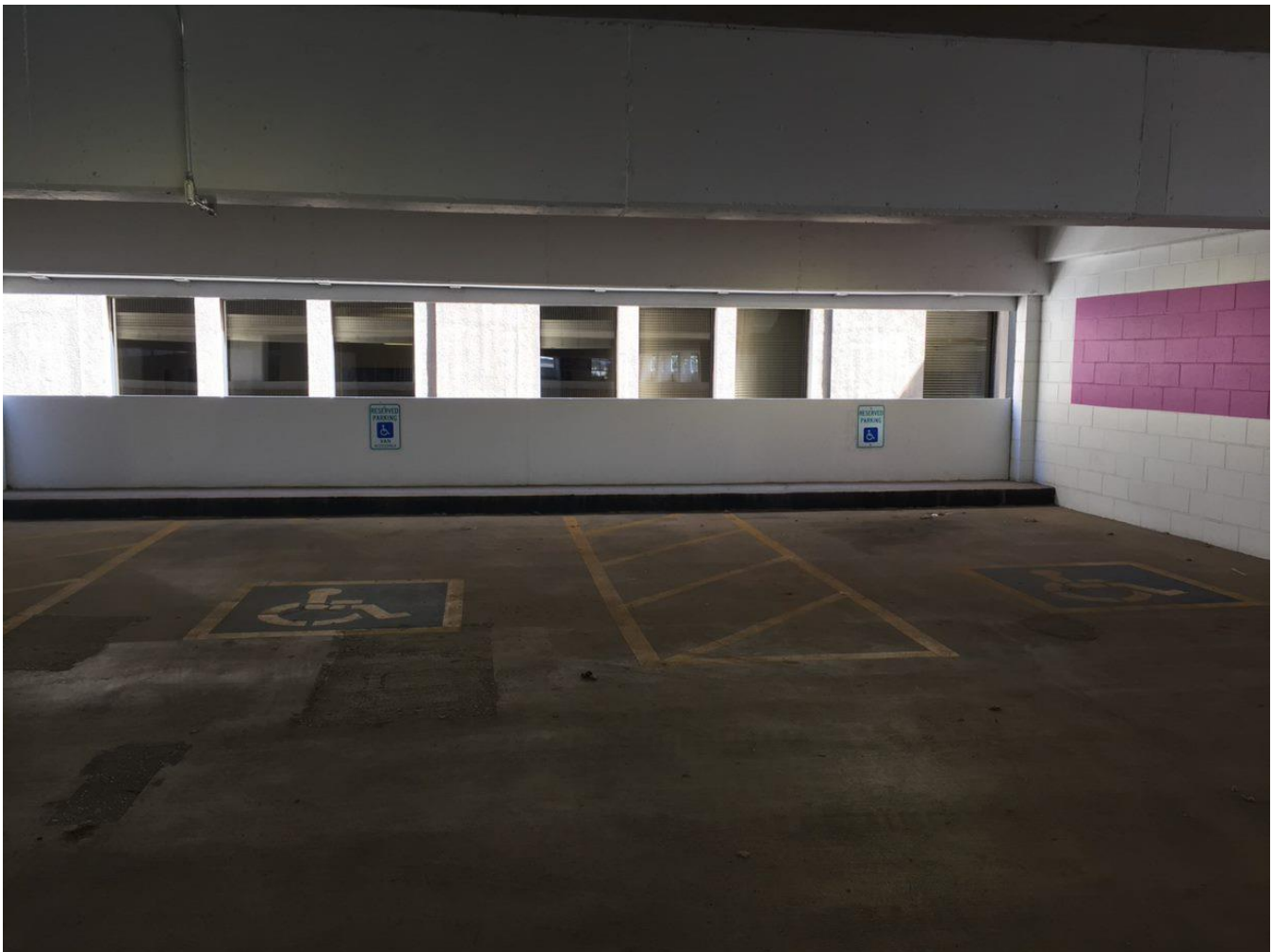
Exhibit 9: Sheridan and Walker Parking Structure Van Accessible Space – Level 4
