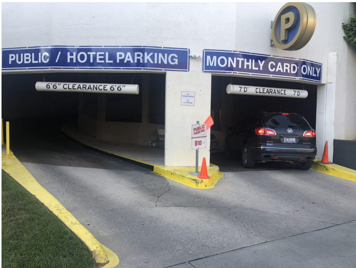
Exhibit 13: Century Center Parking Structure – Sheridan Avenue Entrance
