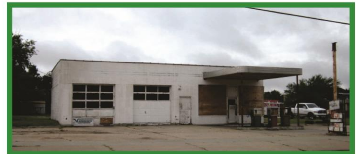
Existing Gas Station
