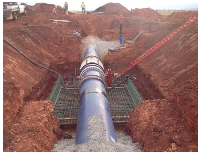
48-inch main extension
