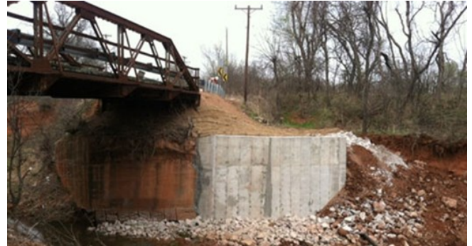
Douglas Boulevard Bridge
