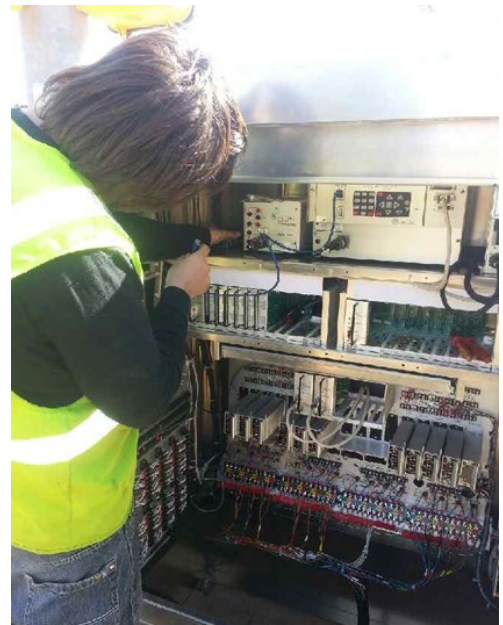
ITS Controller Installation
