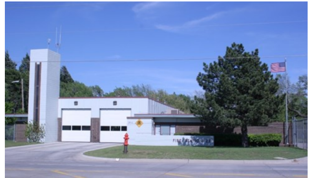
Station 23 to be Re-built
