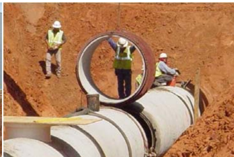
At left is construction at the Chisholm Creek Wastewater Treatment Plant. Above, wastewater pipes are being laid.
