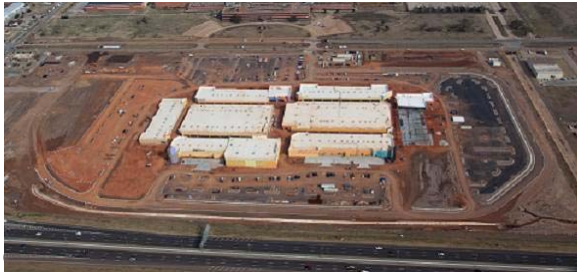
An aerial view of the new outlet mall presently under construction.
