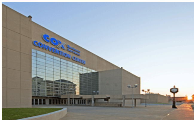
Cox Convention Center renovations were recently completed.
