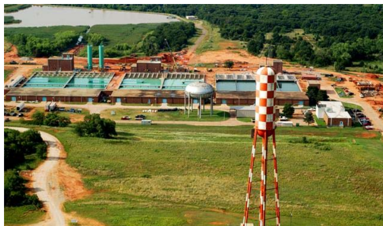
Lake Hefner Water Treatment Plant
