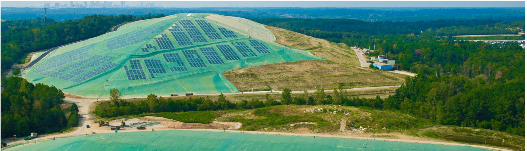
ABOVE: HICKORY RIDGE LANDFILL IN ATLANTA, GEORGIA
