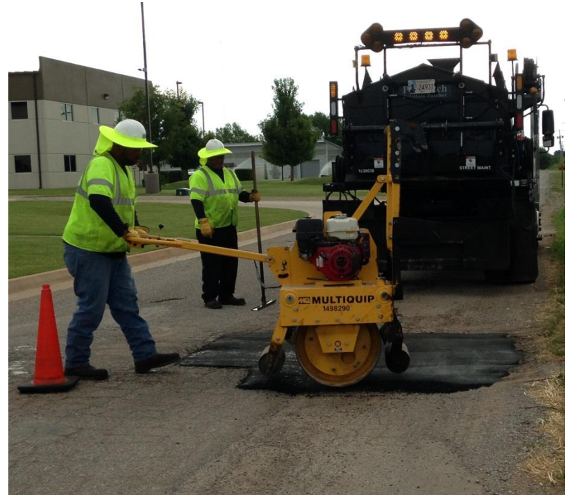
Asphalt Compaction
