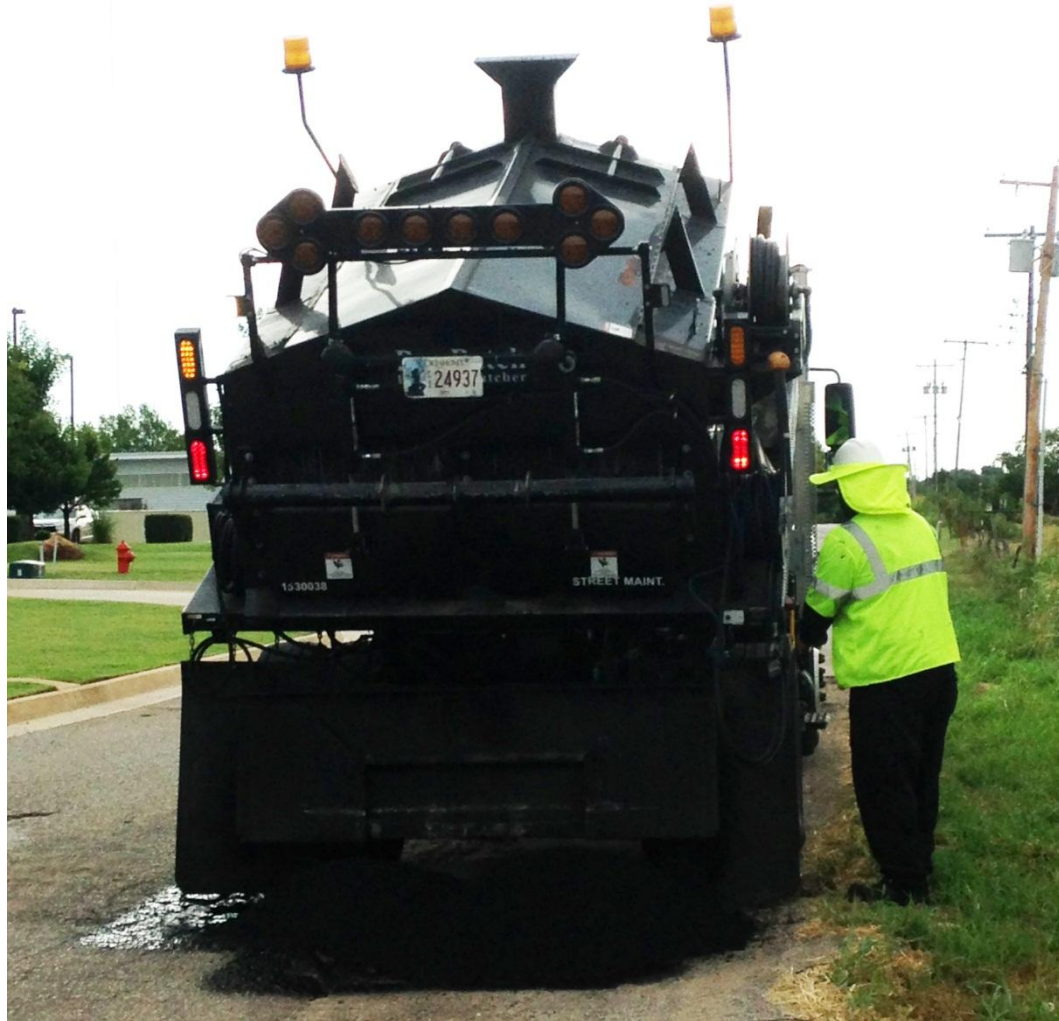
Asphalt Placed in Pothole
