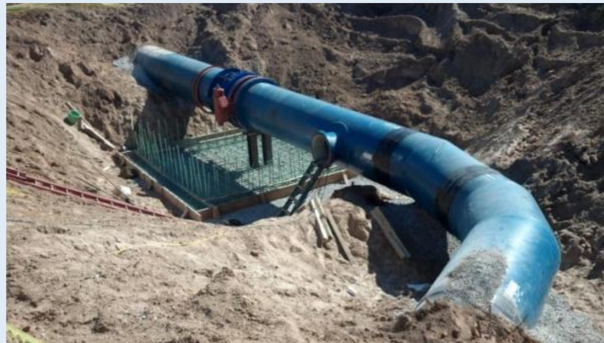
48-inch water main extension
