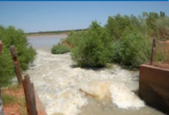
Atoka pipeline outlet at Draper Lake
