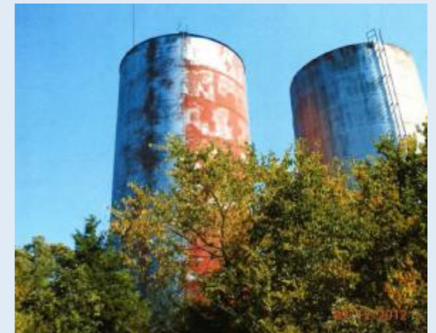
Existing Atoka surge control towers
