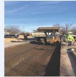
roadway pavement removal
