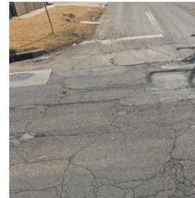
SW 15th Street - Before and After
