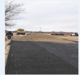
roadway base layer installation
