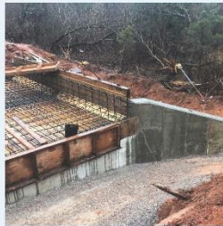
wing walls and steel forms
