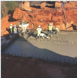
placing concrete floor of structure
