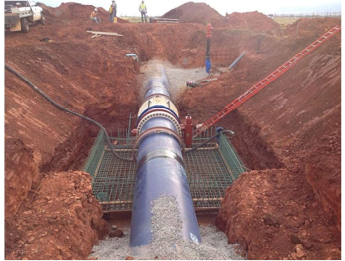
48-inch main extension
