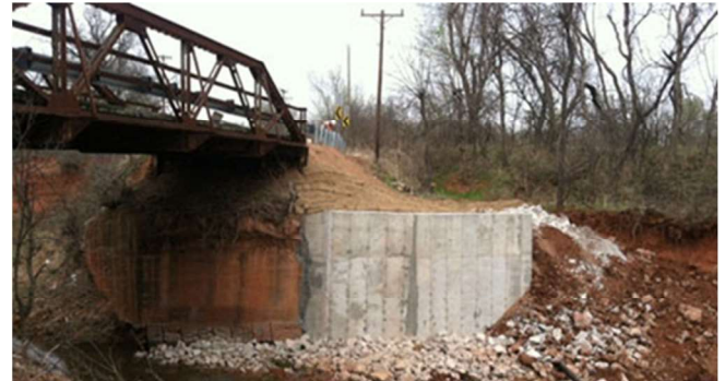
Douglas Boulevard Bridge
