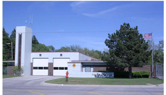
Station 23 to be Re-built
