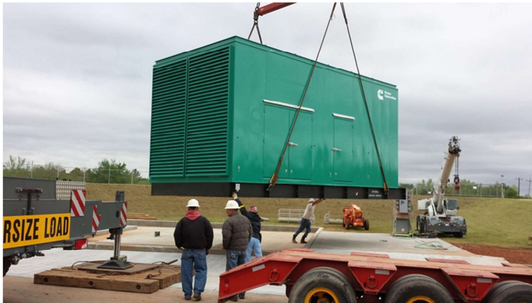
Witcher Lift Station Generator
