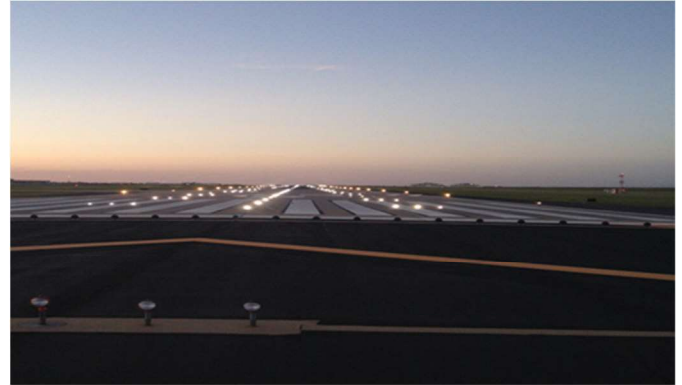
Airport Lighting Control and Movement System
