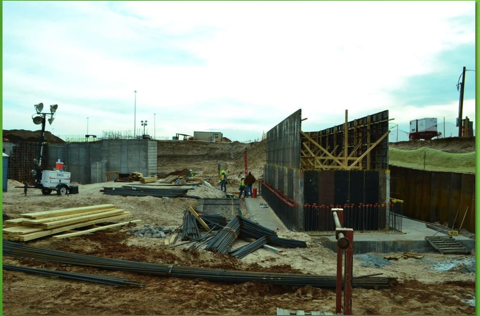
Conveyor Inlet Structure- March 17, 2015
