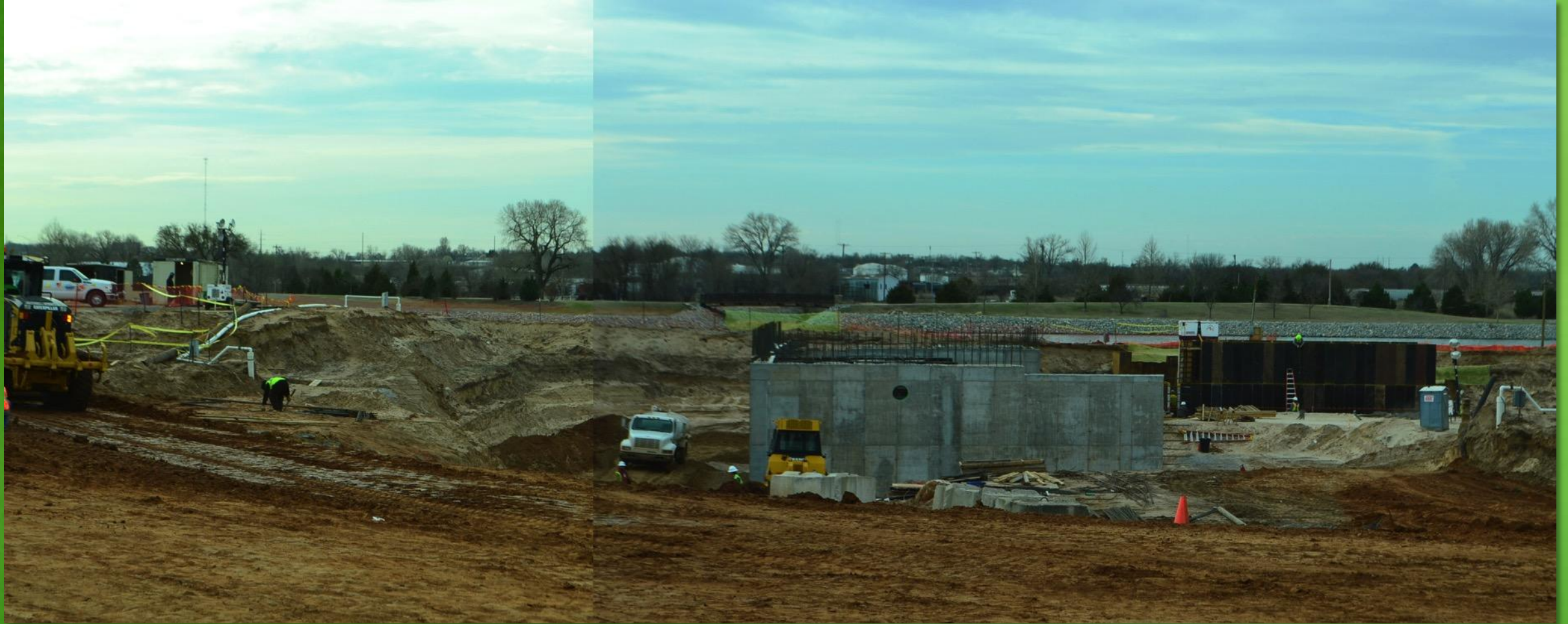
Looking South, Pump Station and Upper Pool- March 17, 2015
