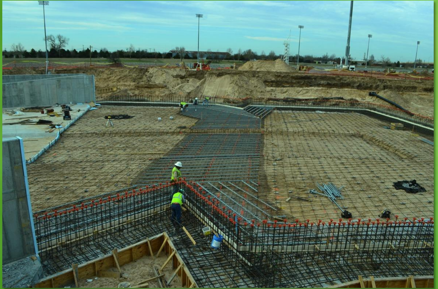
Bottom Pool 4 th Slab Pour, 1 st Unistrut- March 17, 2015
