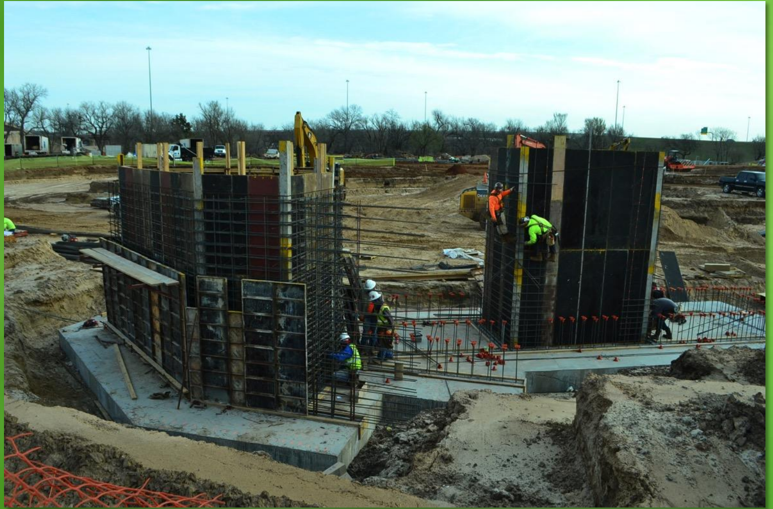
Pedestrian Bridge Abutments- March 17, 2015
