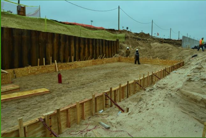
Conveyor Inlet Structure- February 20, 2015
