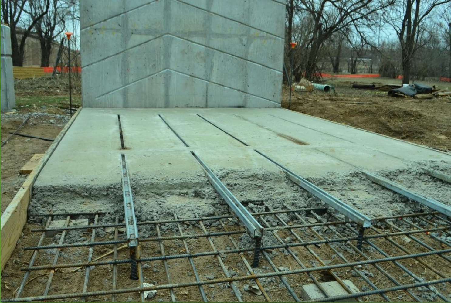
Finishes- Unistrut Test Panel – February 20, 2015
