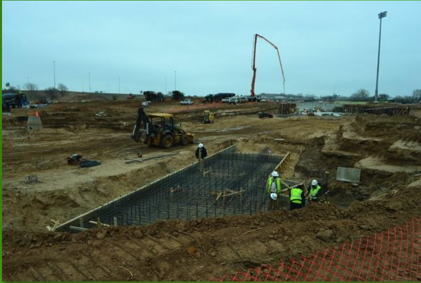
Pedestrian Bridge Abutments- February 20, 2015
