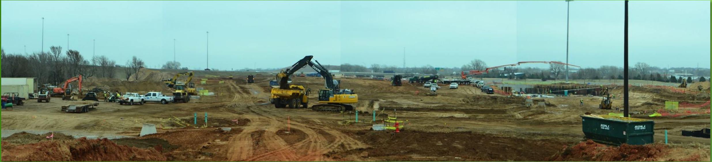
Looking Southeast, Channel Wall Pour– February 20, 2015
