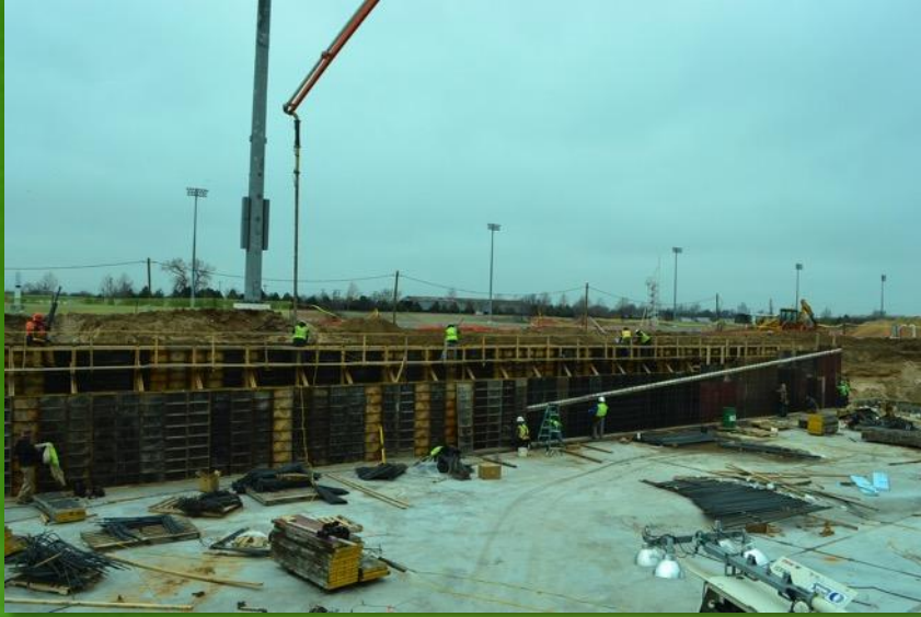
Channel Wall at Ramp– February 20, 2015
