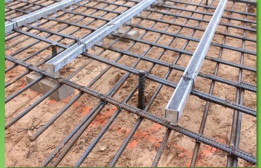
Bottom Pool 4 th Slab Pour, 1 st Unistrut- March 17, 2015
