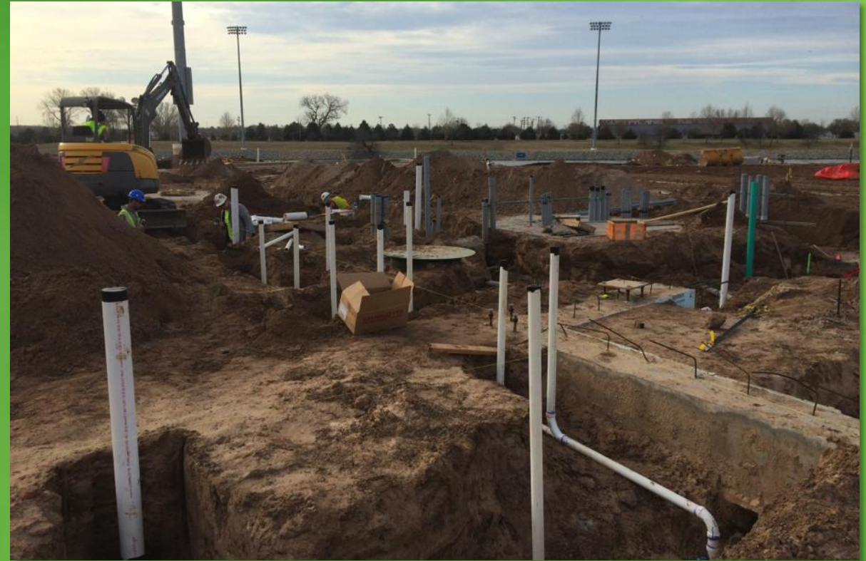
Main Building Under Slab Rough-In– March 17, 2015
