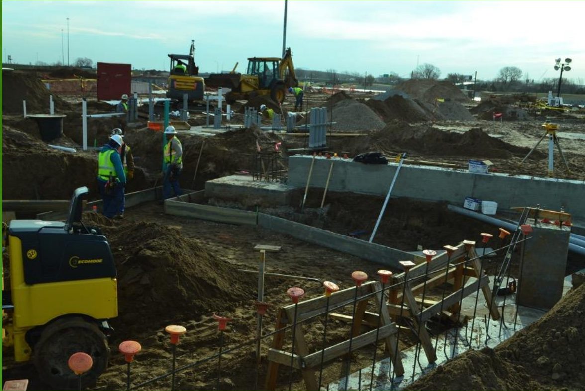
Main Building Under Slab Rough-In– March 17, 2015
