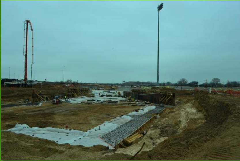
Bottom Pool 4 th Slab Pour, 1 st Unistrut- February 20, 2015
