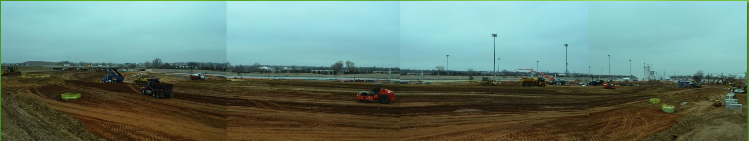
Looking South, Recreational Channel Import– February 20, 2015
