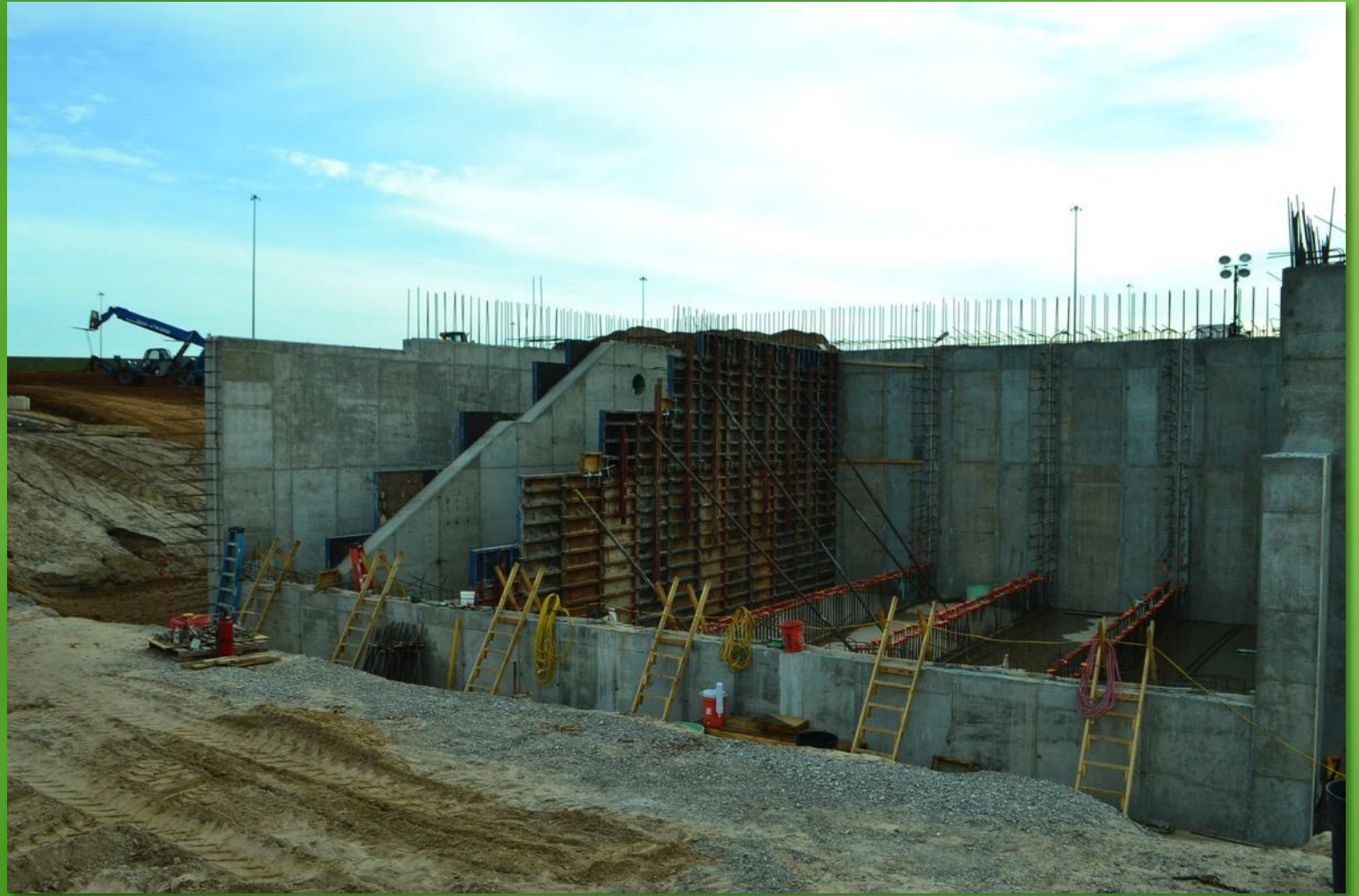
Pump Station- March 17, 2015
