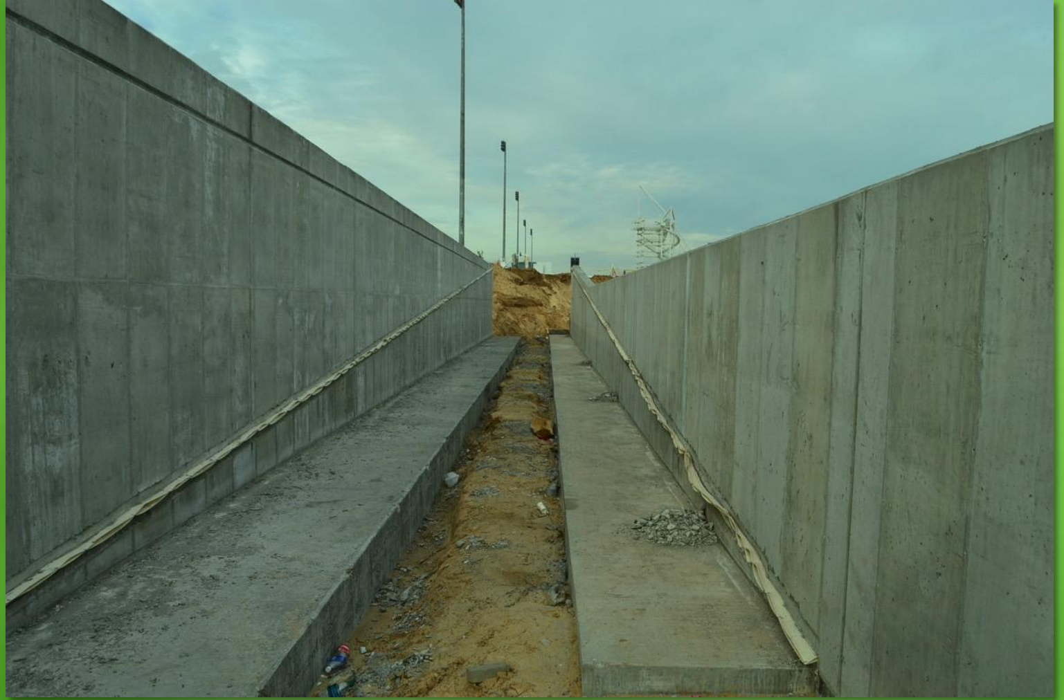
Channel Wall at Ramp- March 17, 2015
