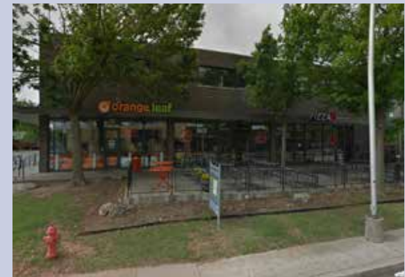
Existing building with parking in the back abutting residential lots. Ground floor frontages result in better connection to street.
