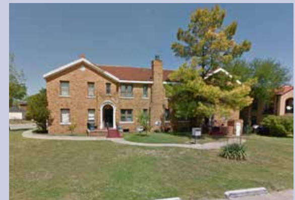
Existing house-scale multifamily with small parking court at the rear of lot and common open space.
