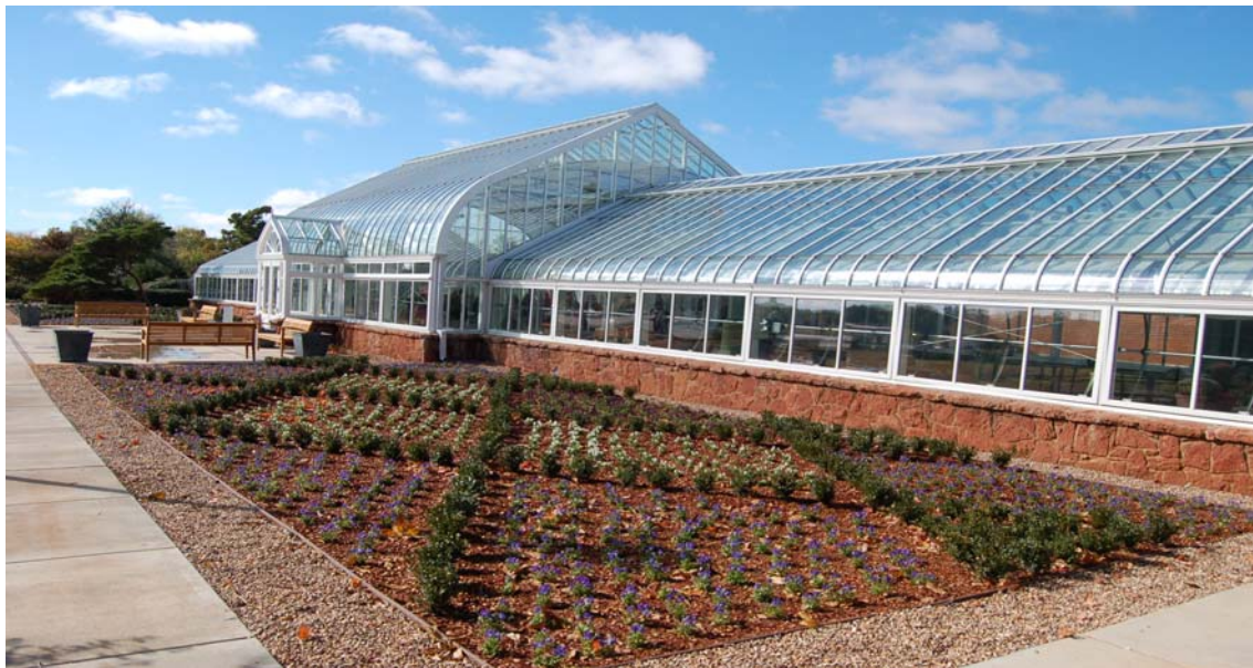
Renovated Lycan Conservatory at Will Rogers Gardens Paid for by 2007 General Obligation Bond Funds
