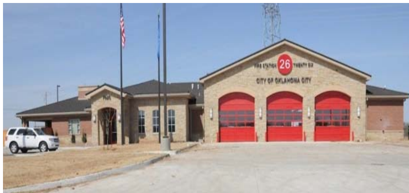
New Fire Station #26 located at 7025 SW 119th St. Paid for with General Obligation Bond Funds.
