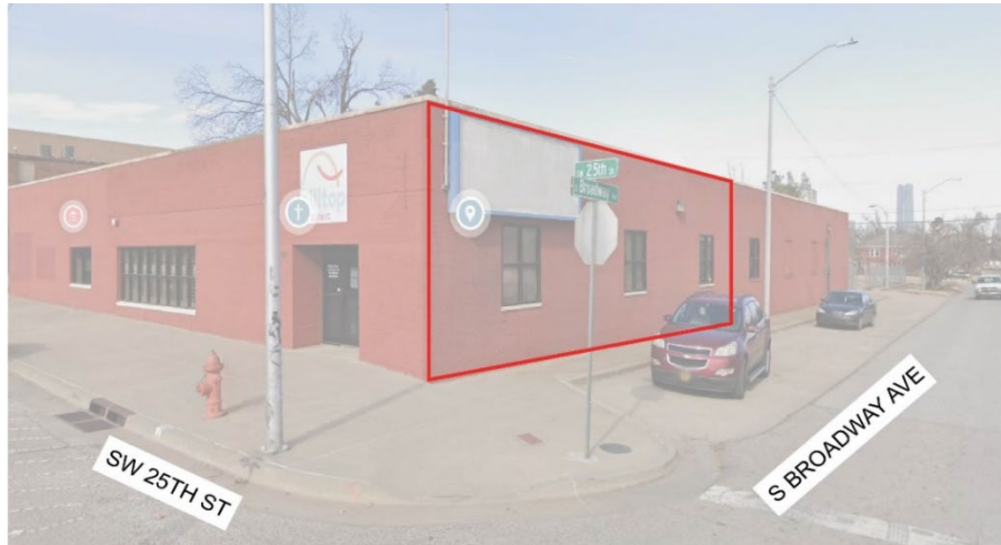
Figure 1: Mural Location. Highlighted in red is location for public art. Wall faces east.
