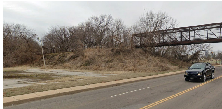
Katy Trail / NE 10 th Street View looking SW
