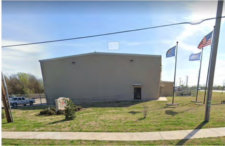
I-1- Light Industrial –all inside
