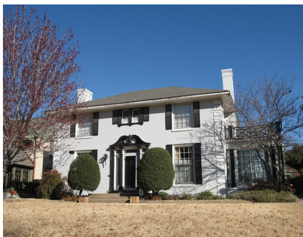
Colonial Revival style dwelling at 1815 NW 40th Street.
