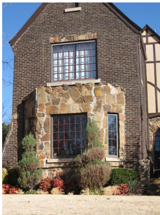
Design guidelines stress the need to preserve original materials that illustrate style and character such as the stone and brick exterior and original windows on the dwelling at 805 NW 40th Street.
