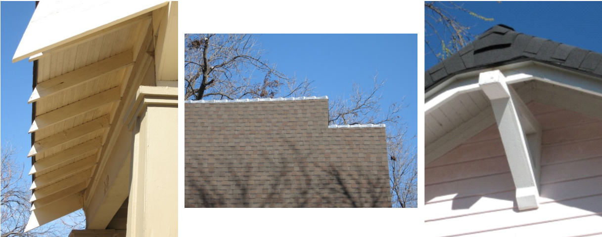
Preserve original related roof features such as rafter tails (left: 2612 N. Hudson), roof ridge tiles (center: 905 NW 38th Street), and brackets, also called knee braces (right: 1442 NW 37th Street).
