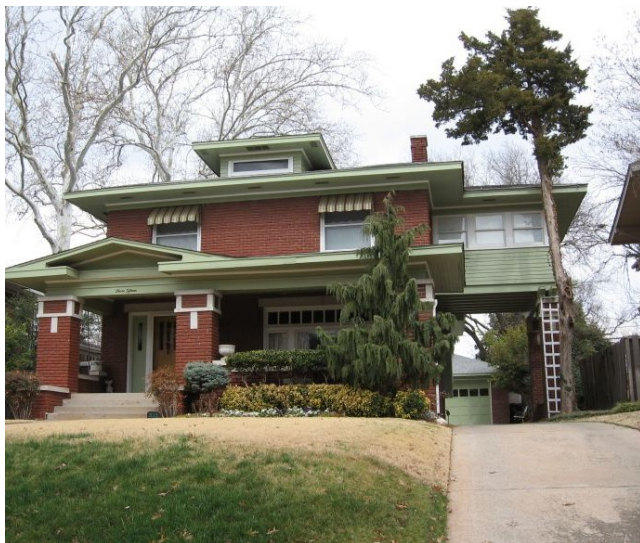
The porte-cochere at the end of the driveway at 315 NW 17th Street is an important character defining feature of the building.
