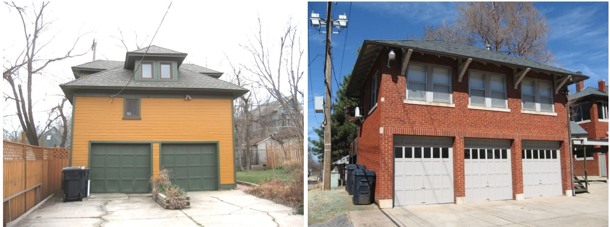
The original garages at 610 NW 17th Street (left) and 2601 N. Hudson Street (right) observe the traditional setback for secondary buildings, which is to the back of the primary building.
