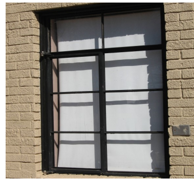
Steel casement windows (left: 801 NW 40th Street and 2240 NW 27th Street, right) can be replaced in-kind, if necessary. Steel window manufacturers offer rust-proof galvanized models in custom colors that may never require re-painting.
