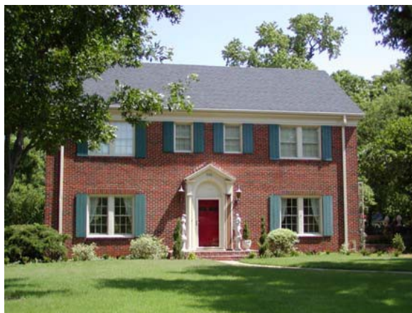
Georgian Revival style dwelling at 1525 NW 35th Street.
