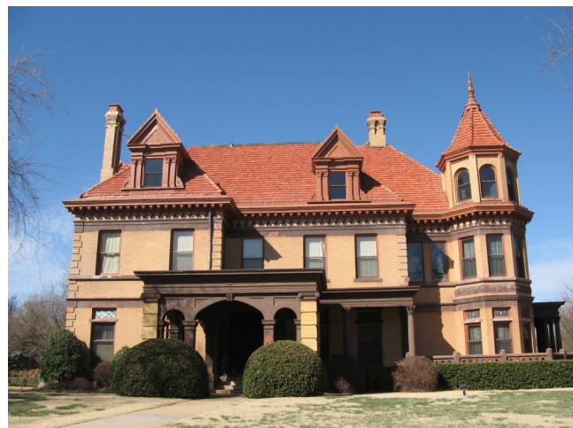
The Overholser House at 405 NW 15th Street is one of Oklahoma City's best examples of the Queen Anne style.
