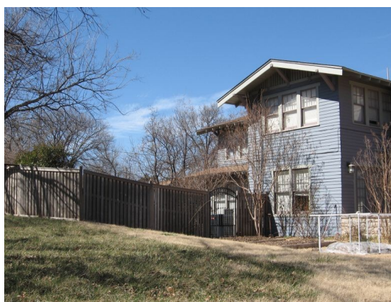
This wood privacy fence at back of 2727 Harvey Avenue is located and designed appropriately.
