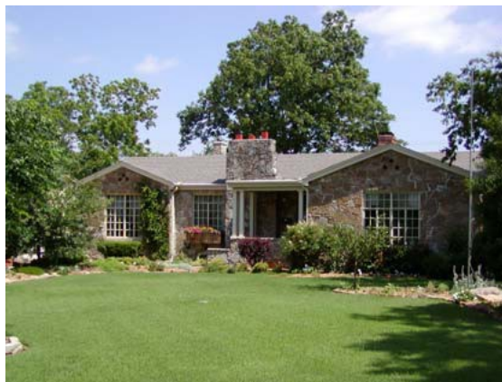
Minimal Traditional dwelling at 1619 NW 38th Street.
