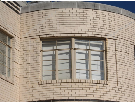
Steel casement windows (left: 801 NW 40th Street and 2240 NW 27th Street, right) can be replaced in-kind, if necessary. Steel window manufacturers offer rust-proof galvanized models in custom colors that may never require re-painting.
