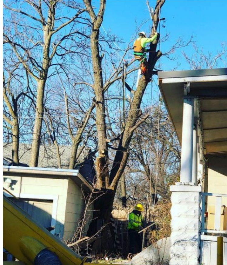
Hazardous tree trimming & removal
