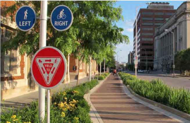
Bicycle facility built off of the traffic zone and into the pedestrian zone
