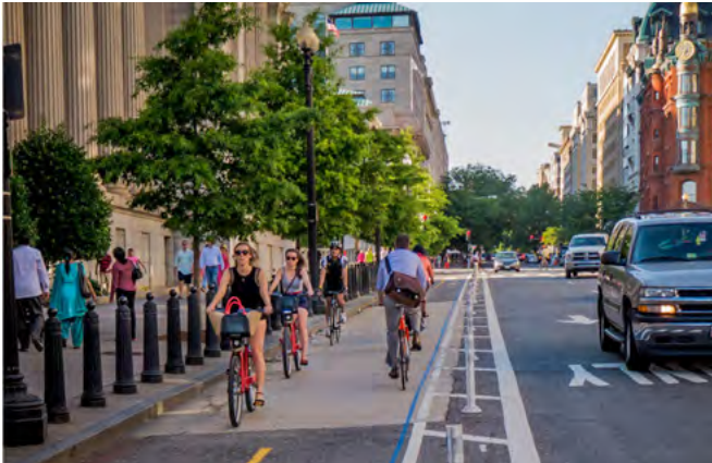
Designated bicycle lane adjacent to curb, separated by large buffer zone which may include physical barriers like bollards or low walls. Can be one-way or two-way / contra-flow. Lane is in-between parking and the curb.
