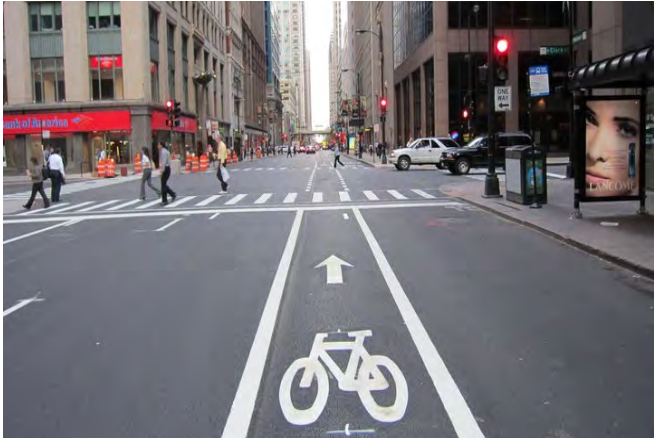
Delineated lane for cyclists, 4+ feet wide with solid white line separating bicycle lane from traffic or parking. Lane is typically in-between traffic and parking lane.
