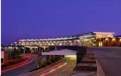
AIRPORT BRIDGE DECK REHABILITATION
