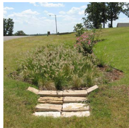
Bioretention cell retrofit
