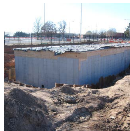
Construction of new sand filter
