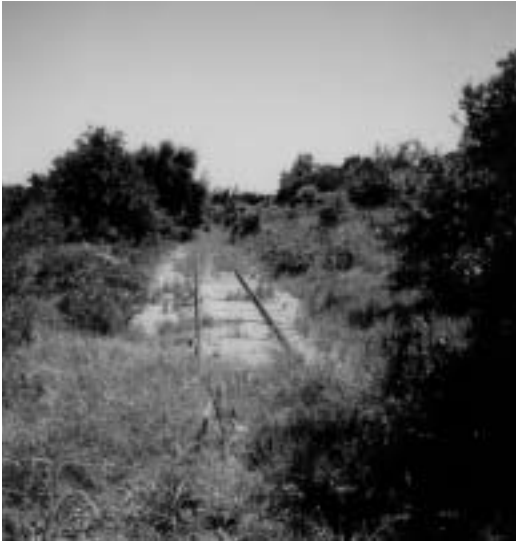
The Katy Trail would utilize an abandoned railroad corridor
