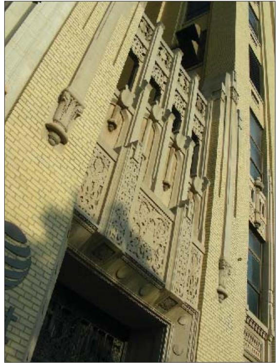
Gradual weathering can subtly enhance masonry texture and detail.
