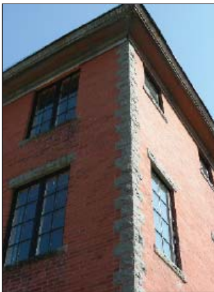
Retain the traditional relationship and profile of window frame to wall surface.
