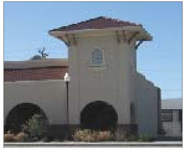
Corner emphasis using roof form.
