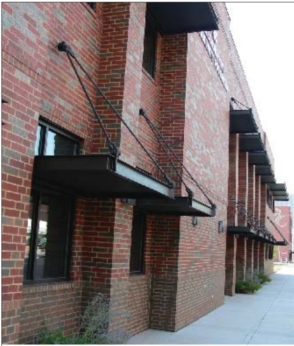
Traditional elements, such as canopies, can be effective additions in energy management.
