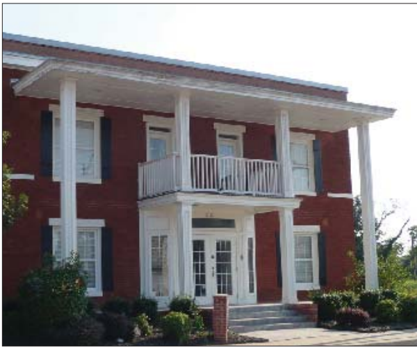
Retain original wood and repair if it becomes necessary.
