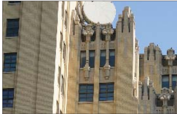
Position service equipment away from public view. Here, the dish detracts from the character of the building.
