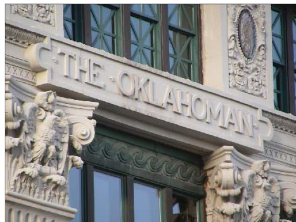
Masonry can be carved or cast to create association and individuality in classical detailing.
