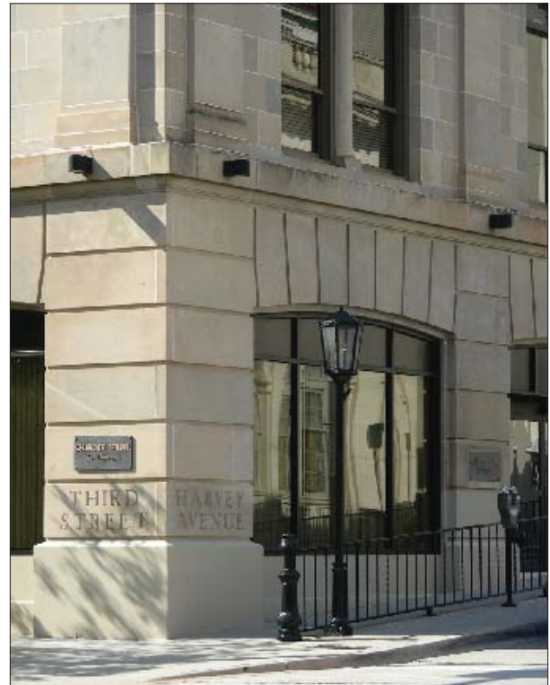
Architectural lighting can be discreetly designed and placed, such as those on the molding of the building.
