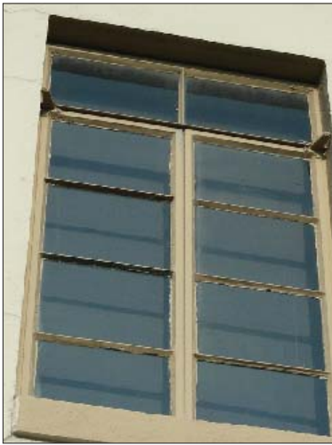
Traditional steel casement frames are durable as well as characteristic.
