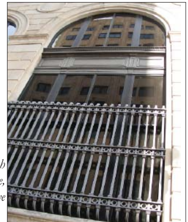
Metalwork can embellish the facade as window frame, spandrel, and decorative railing.
