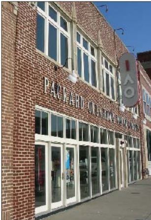
External traditional lighting can enhance the street facade.
