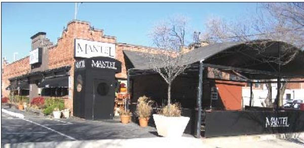
An alteration should be designed to avoid damage to the original building. This canopy, for example, is reversible and does not damage key features of the building.
