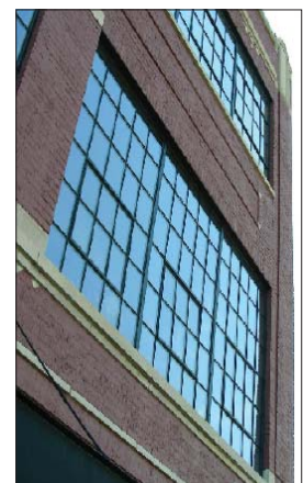
Traditional steel frames with opening lights are characteristic of many buildings.
