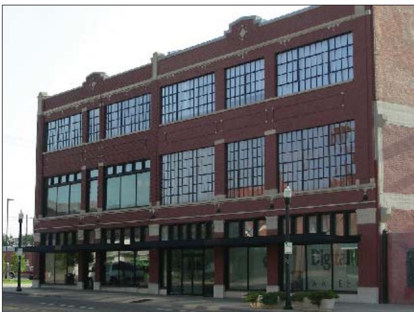
The 'solid to void' relationship of wall to window is a primary characteristic of a building.
