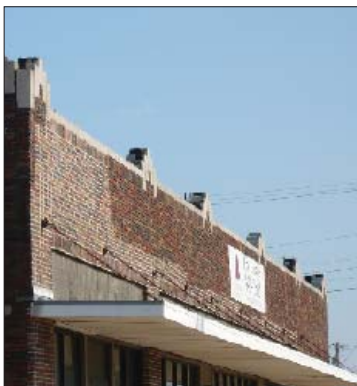
A traditional canopy distinguishes between storefront and parapet detail.
