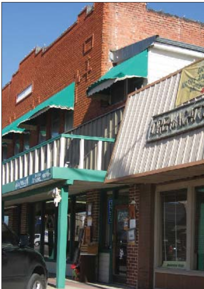
Avoid painting brickwork that has not been painted.
