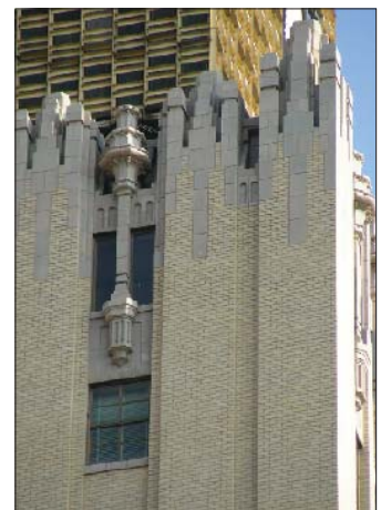
Parapet in the form of pinnacles.
