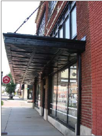
The canopy provides distinctive detailing appreciated at street level.
