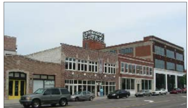
Traditional lot widths create a framework for architectural richness and urban character.
