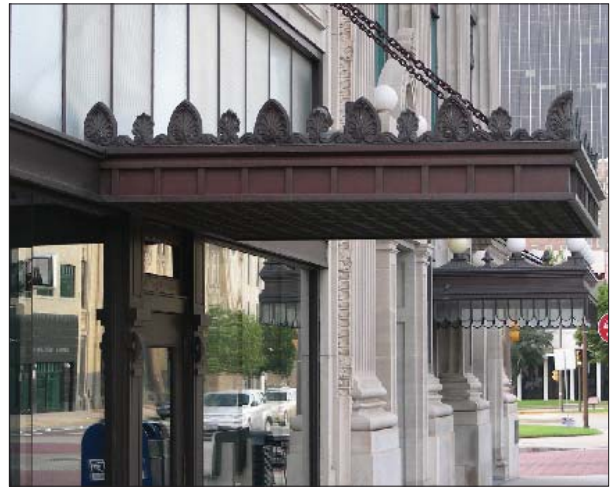
A traditional entrance canopy is usually legible, functional, and decorative.
