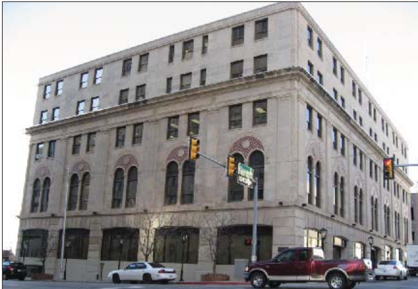
Vertical and horizontal window alignment is central to the facade composition.
