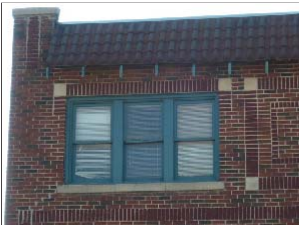
Traditional windows in an upper story are often in the form of sash frames.
