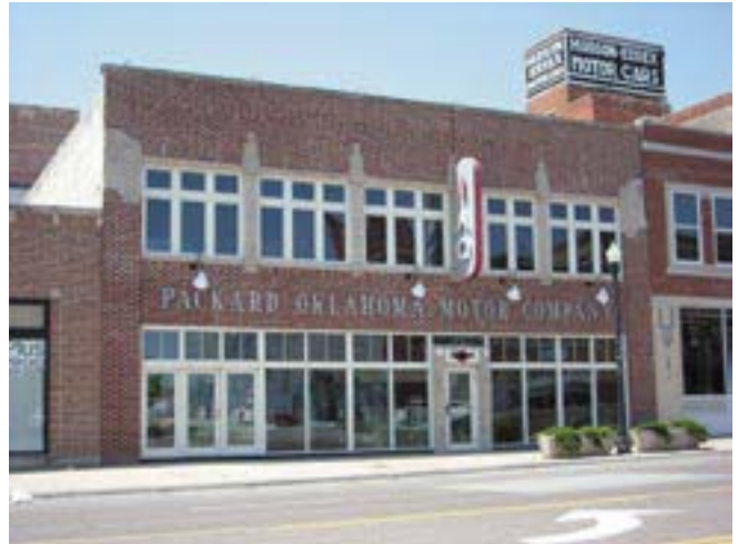
Known for its warehouse / loft conversions, above is one example. Similar to others in the District, the first floor contains retail, with office space occupying the 2nd floor.
