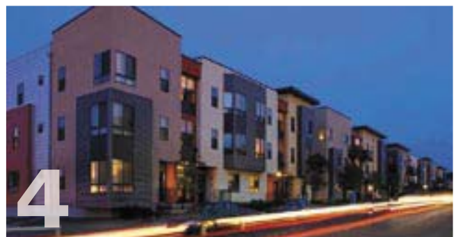
The sample housing development used for the gap analysis included a 3 story, wood frame structure built on a half block site with structured parking. A site plan (1) and representative photos (2) (3) and (4) illustrate what such a development might look like.
