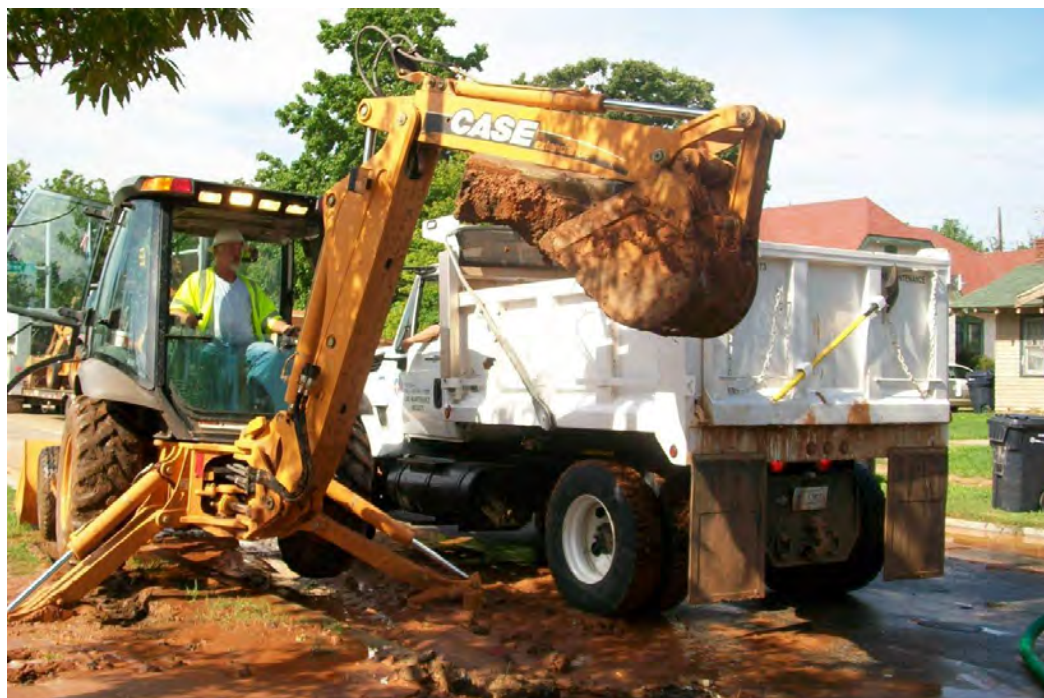
Line Maintenance employees repair a water line.
