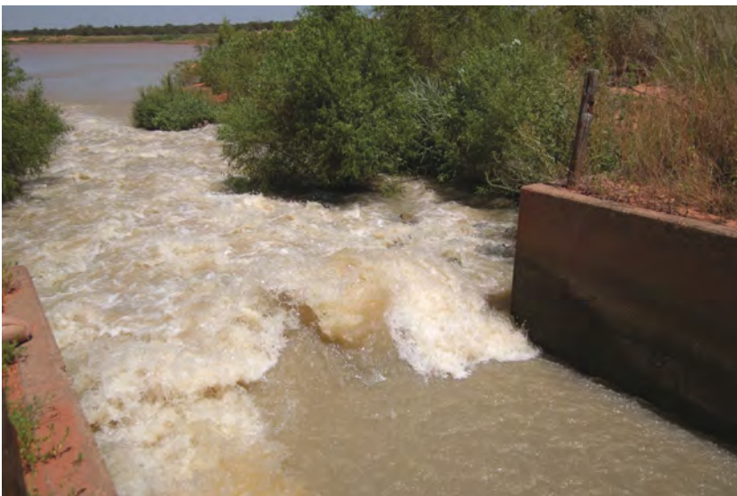
Water flows into Draper Lake after a 100-mile journey through the 60-inch pipeline from Atoka Lake.
