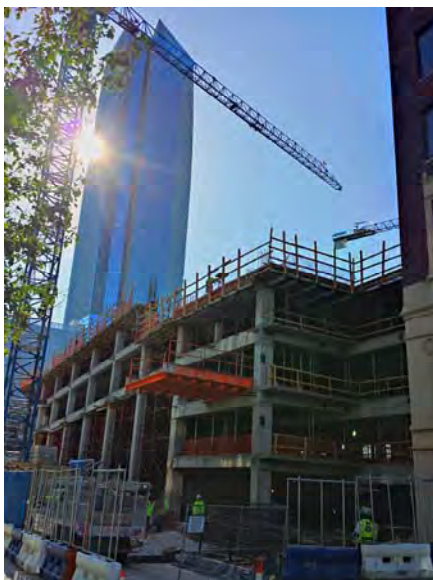
Construction of a parking garage in the Downtown Business District.
