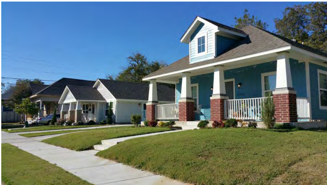
Two new affordable homes in the SNI neighborhood Classen-Ten-Penn. These homes were funded through a federal grant and built by Positively Paseo, a Community Housing Development Organization.
