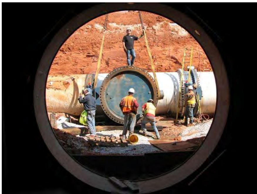
Contract crews install a new 72-inch water line.
