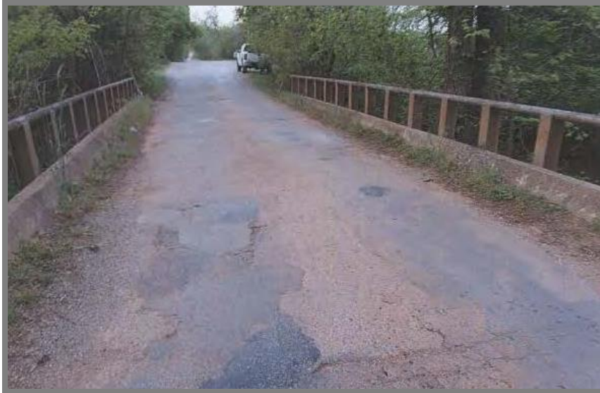
Frisco Road Bridge – south of NW 164th Street
