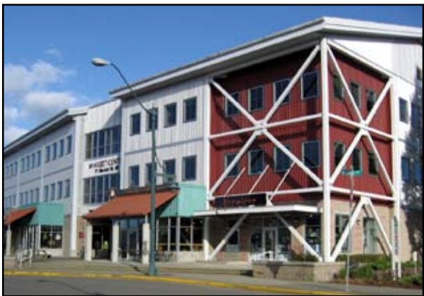
Corrugated metal used as a primary building material. Heavy steel framing used for accent. (Olympia, WA)
