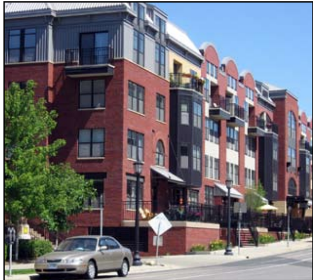
Above and below: Metal used to articulate upper building floors. (Minneapolis, MN)
