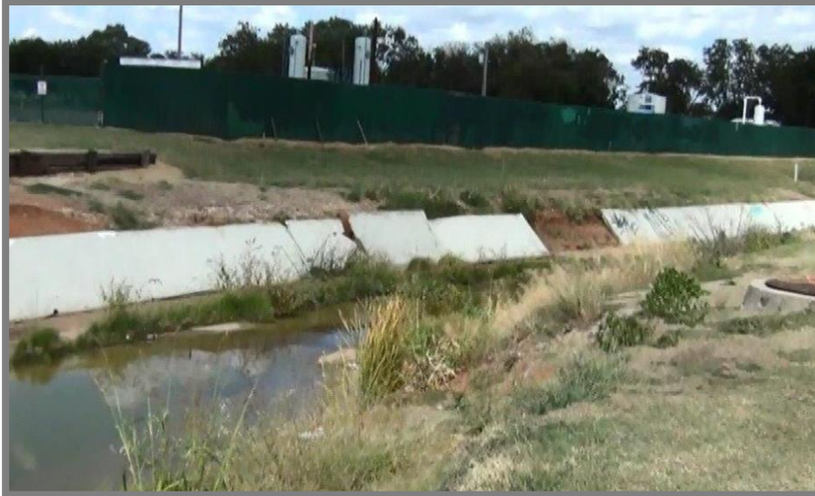
SW 44th Street and May Avenue - Channel Repair
