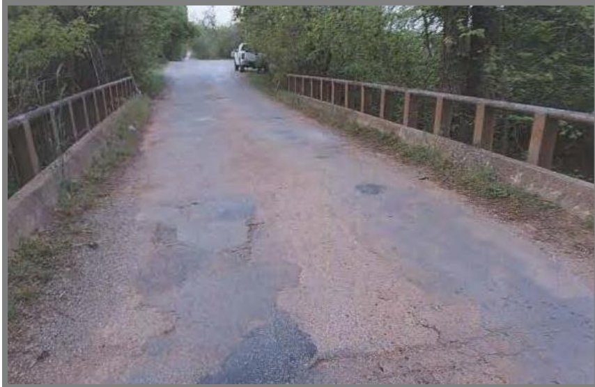
Frisco Road Bridge – south of NW 164th Street
