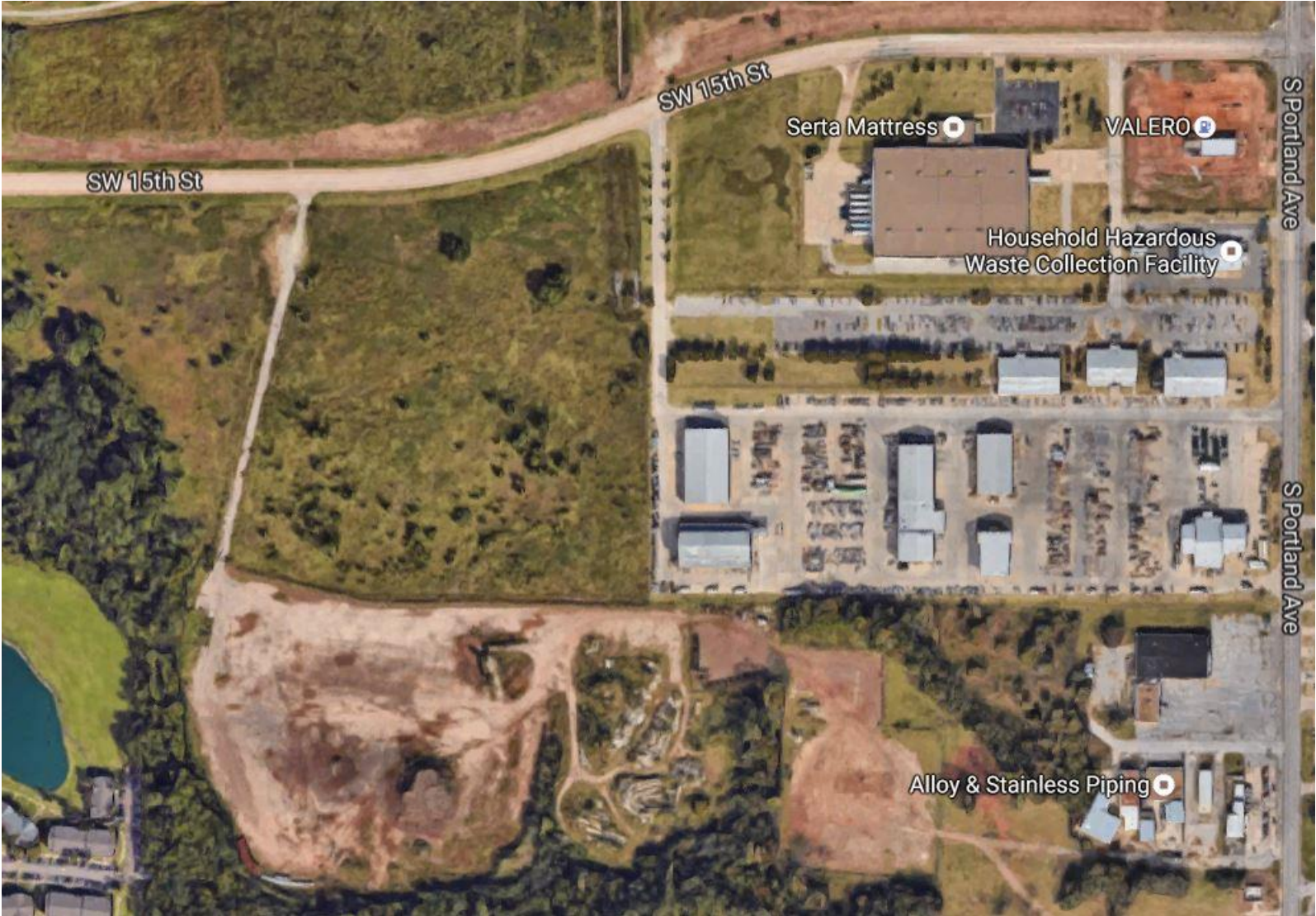
Central Maintenance Facility – 3738 SW 15th Street
