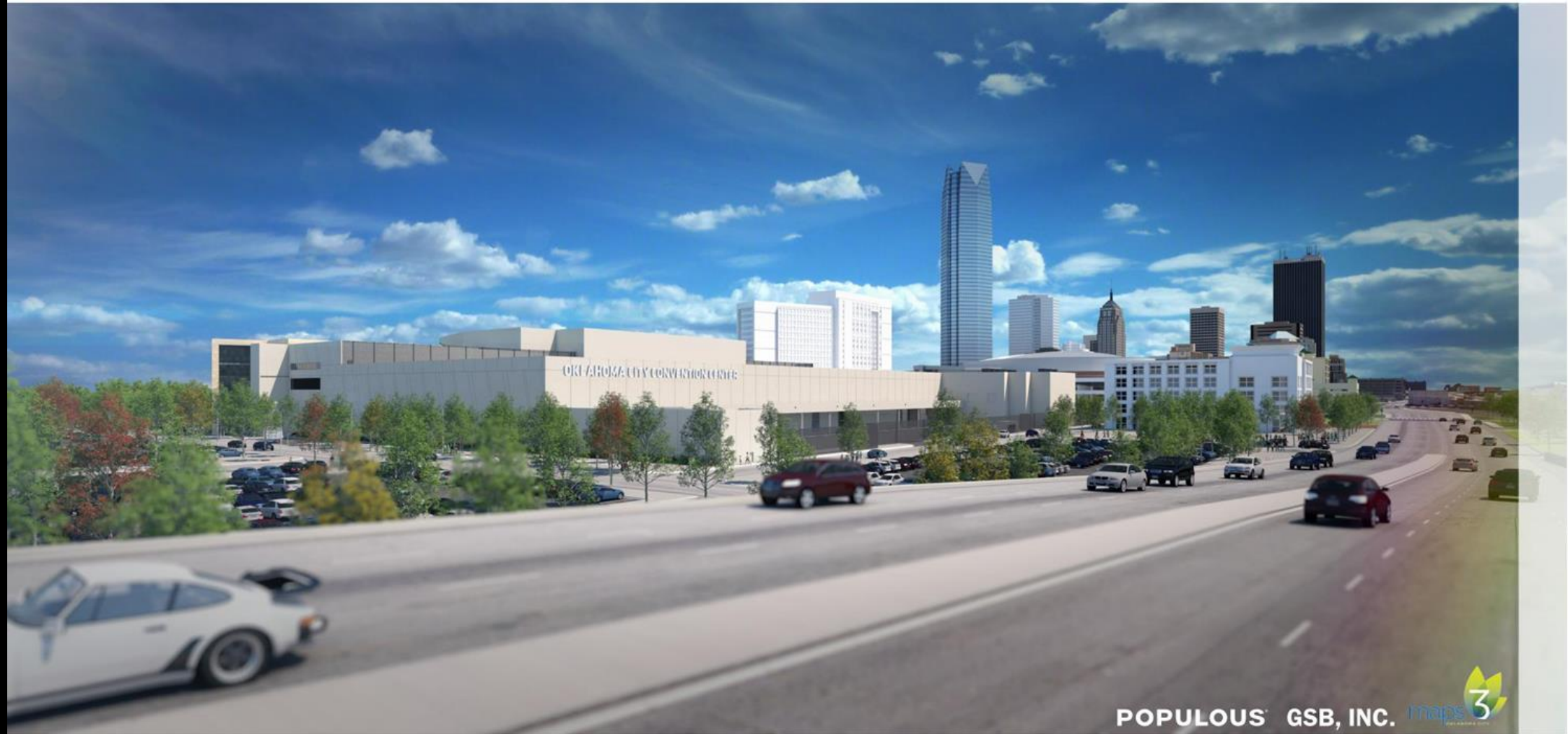
EXTERIOR VIEW - SHEILDS AVE.
