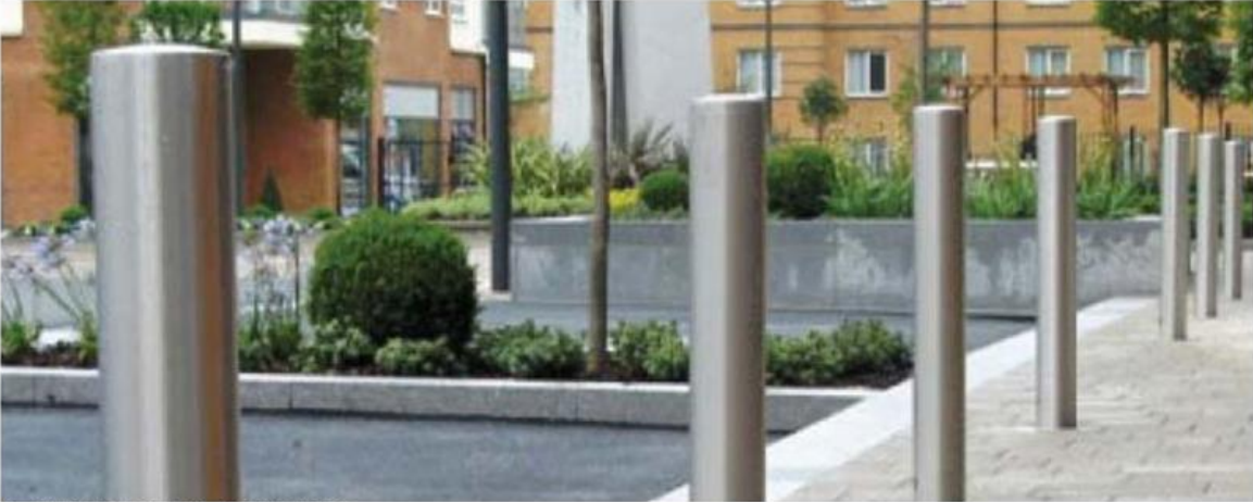
STAINLESS STEEL BOLLARDS
