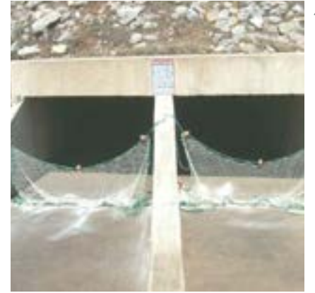
Floatable debris collection nets
