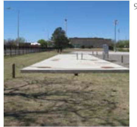
Construction of new sand filter
