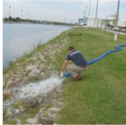
Illicit discharge inspection
