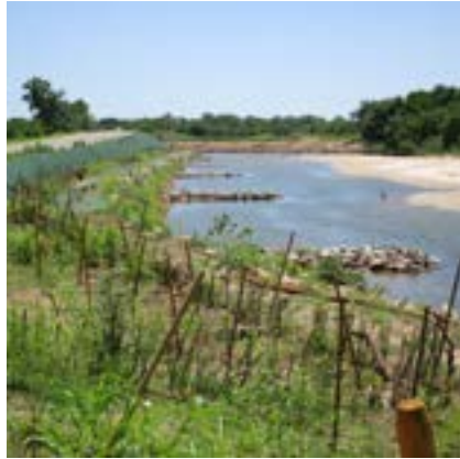
Riverbank stabilization project at Midwest Boulevard and NE 59th Street
