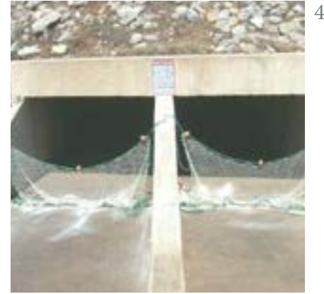
Floatable debris collection nets
