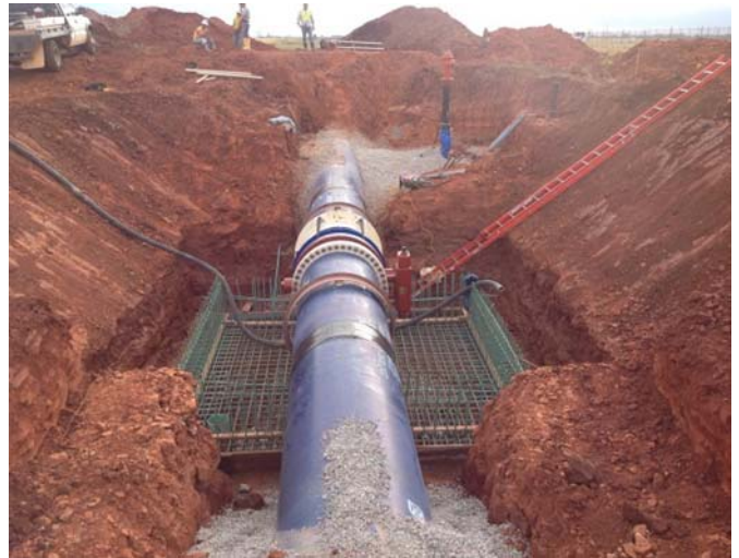
48-inch main extension
