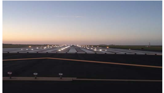
Airport Lighting Control and Movement System
