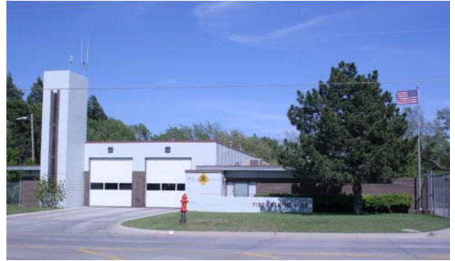
Station 23 to be Re-built
