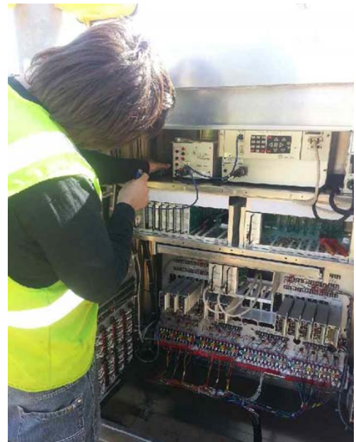
ITS Controller Installation
