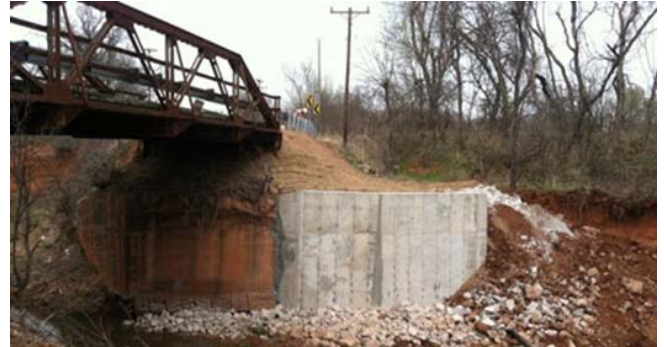
Douglas Boulevard Bridge
