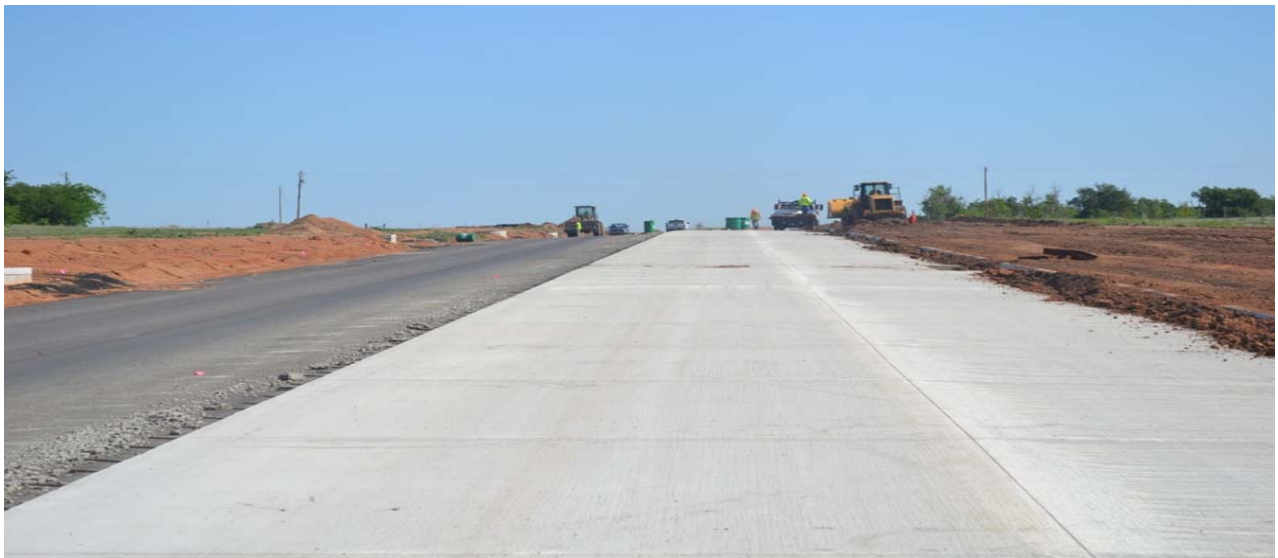
Portland Avenue, SW 74 th St. to SW 104 th St.
