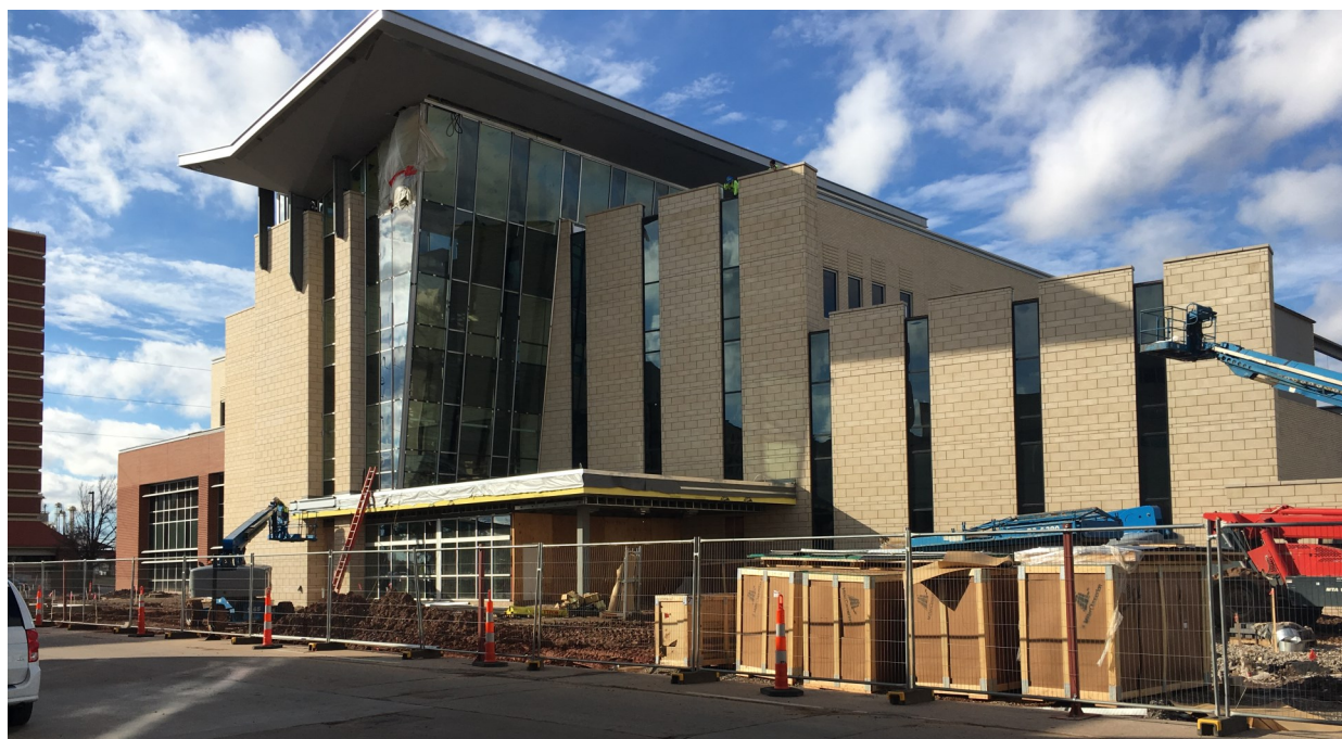
New Municipal Court building under construction
