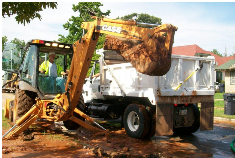
Line Maintenance employees repair a water line.
