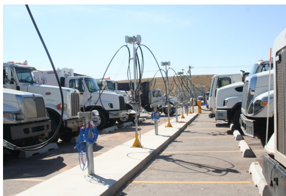
Solid Waste Management trucks refuel at the facility's slow-fill CNG fueling stations.
