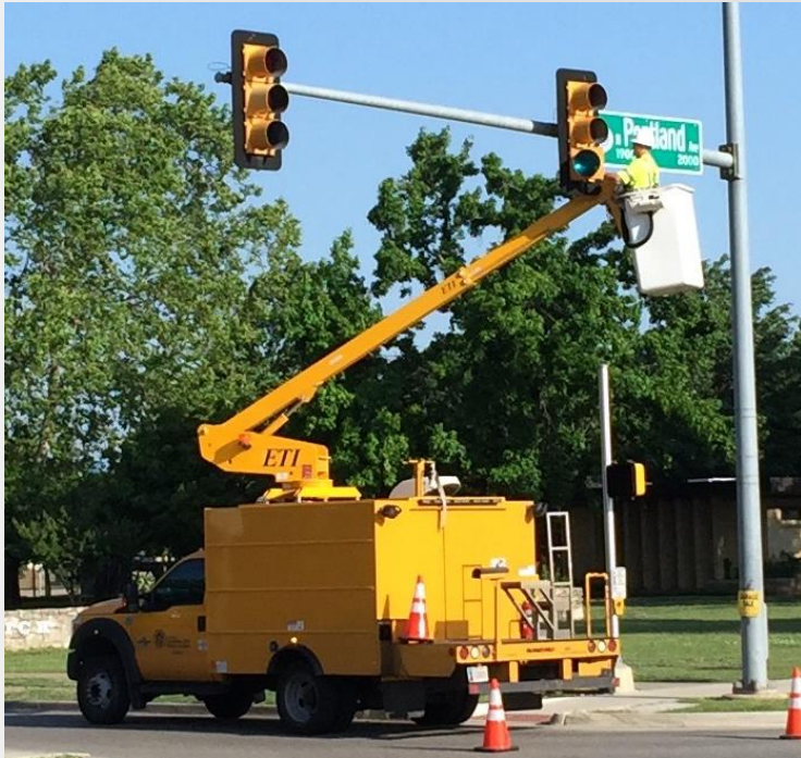
Traffic signal replacement and striping
