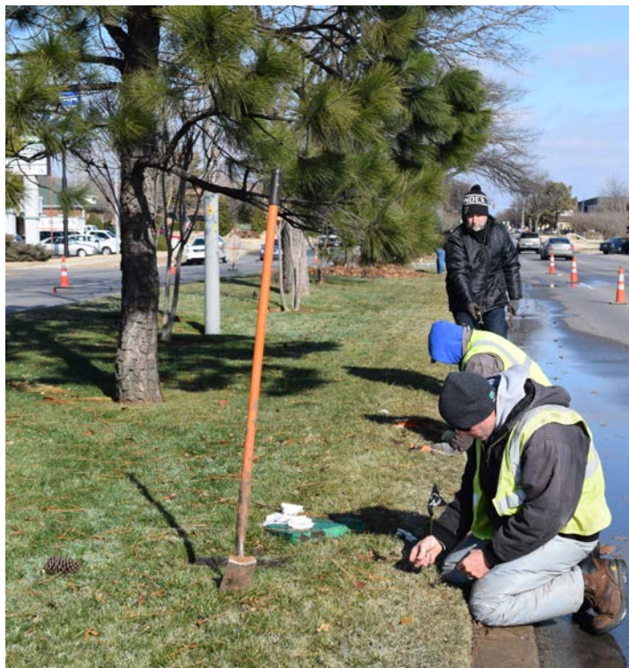
Figure 29: Median retrofit project on Classen Boulevard
