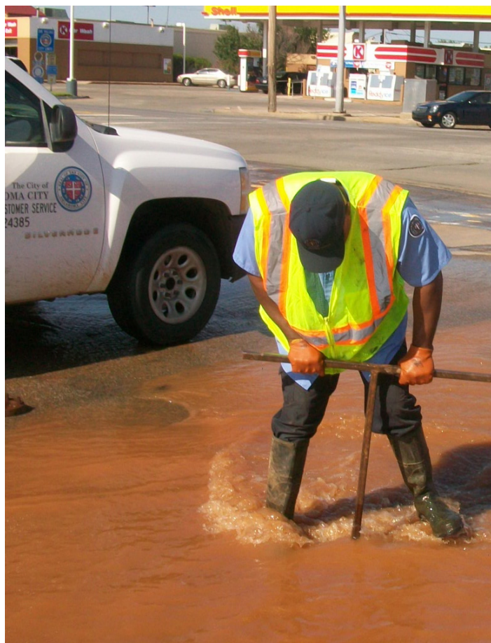
Figure 32: Shutting off water to repair a break
