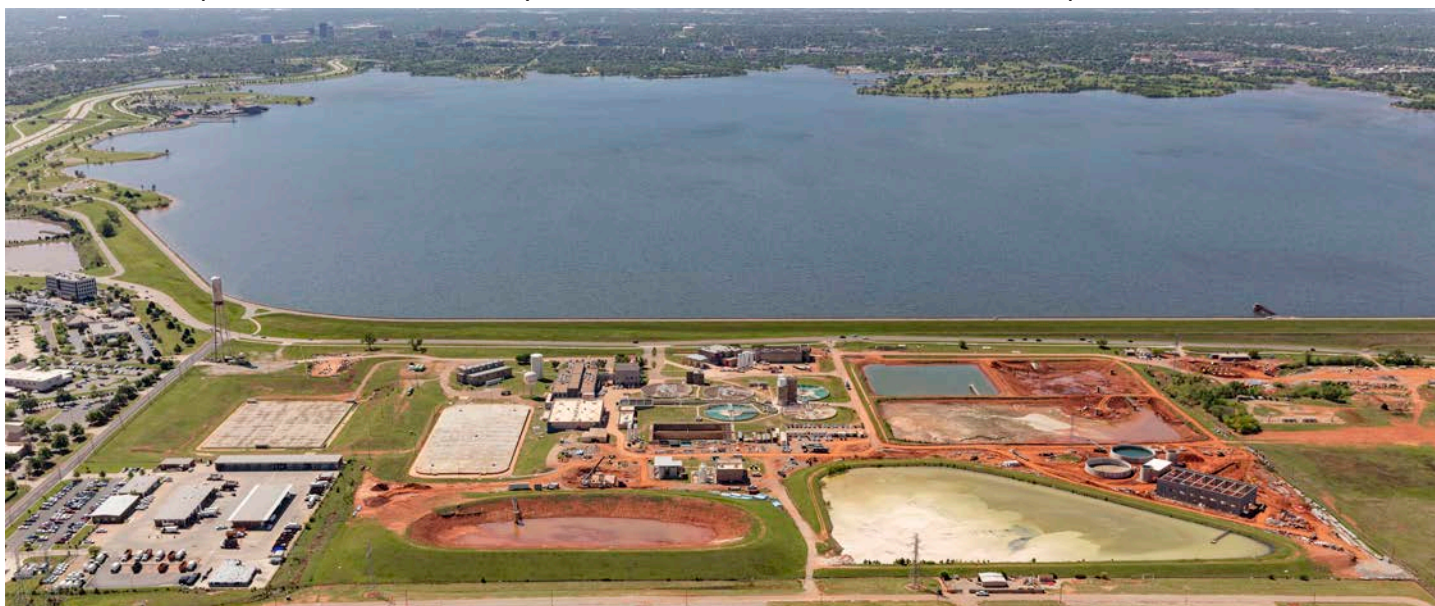
Figure 12: Hefner water treatment plant
